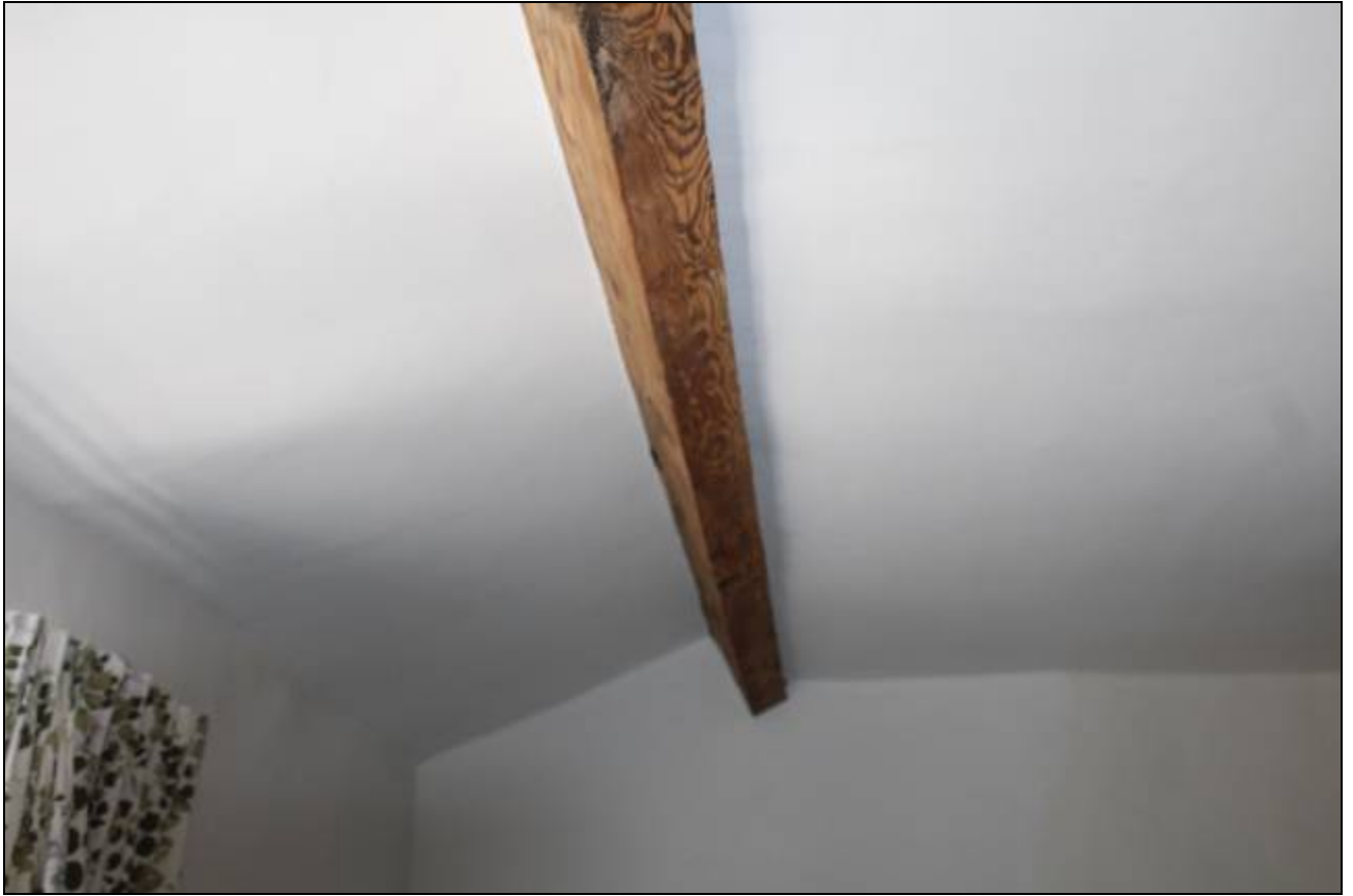
3. Underdrawn ceiling in the third bay bedroom
