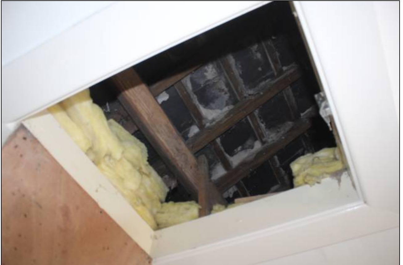
4. View of roof timbers in this room, which have been renewed
