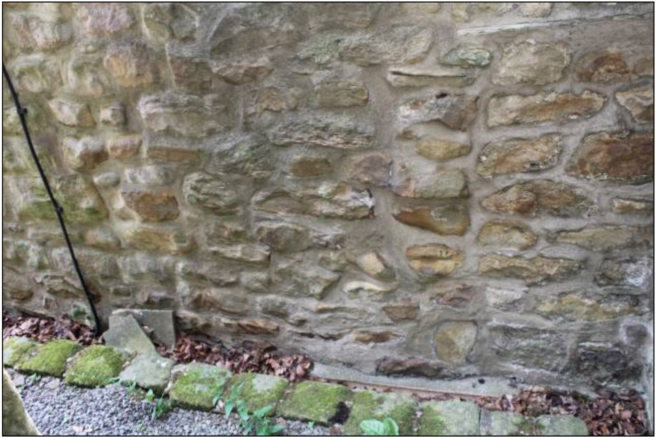
1. The blocked doorway in rear wall of the porch
