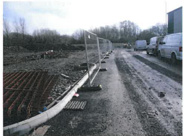
Looking east along the sites southern boundary.
