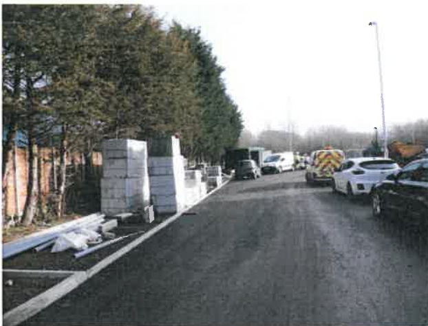
New access road into the site from the west.
