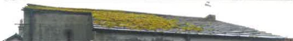
Garage roof has a grey slate finish.
