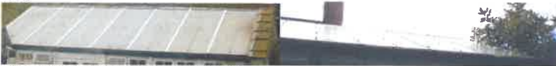
Conservatory roof - Clear upvc sheet with verge stones
