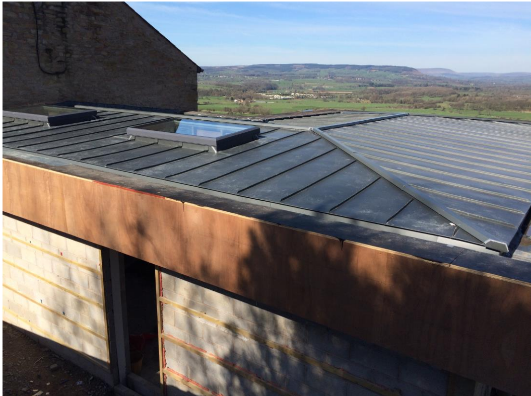
PL02: RheinZink standing seam zinc roof in graphite – grey with Sunsquare Elongated Skyview fixed Flat Roof Skylights.
