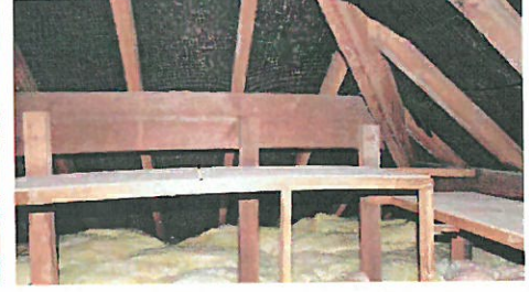
Figure 10: roof void (west)
