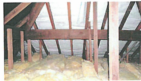
Figure 8: roof void (north)
