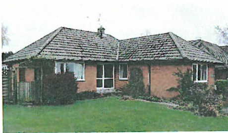
Figure 2: Front / east elevation
