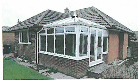
Figure 5: Main roof void
