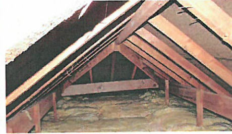
Figure 9: roof void (south)
