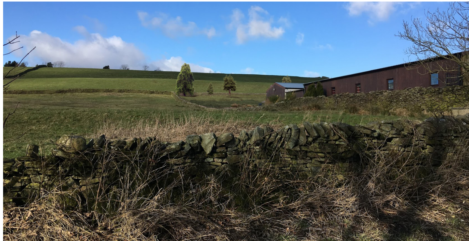
View from within the site boundaries showing the South West elevation of the extended commercial building within the landscaped setting.
