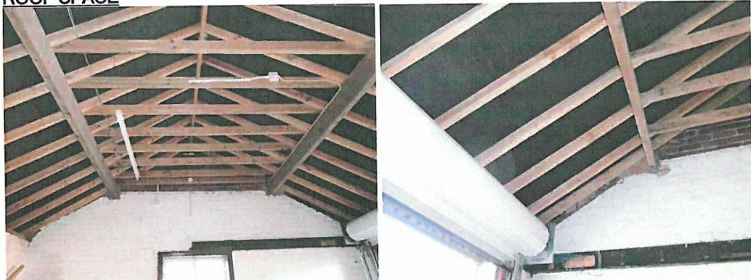
There was no enclosed roof space the timber truss roof structure was easily examined. The felt was in good condition as were the timbers the roof structure did not provide any potential roost habitat.
