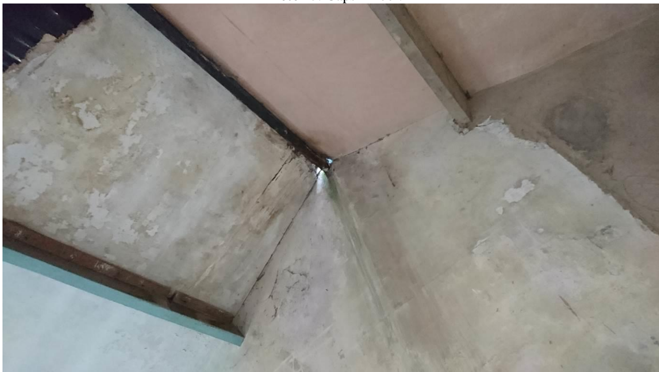
Photo 16: Gaps in internal stonework.
