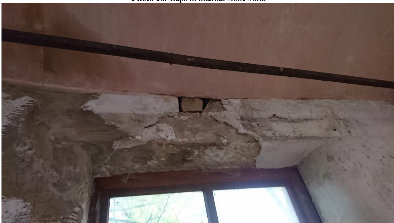
Photo 16: Gaps in internal stonework.
