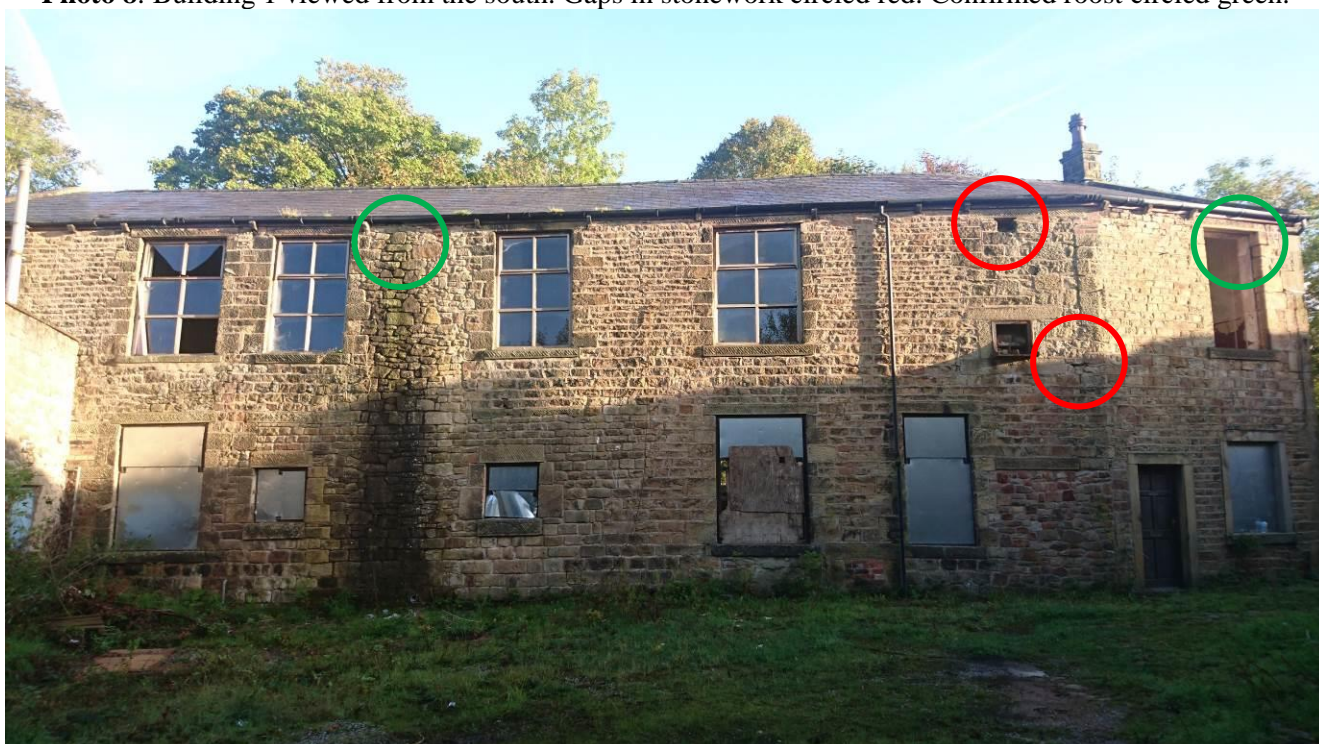
Photo 8: Building 1 viewed from the south. Gaps in stonework circled red. Confirmed roost circled green.
