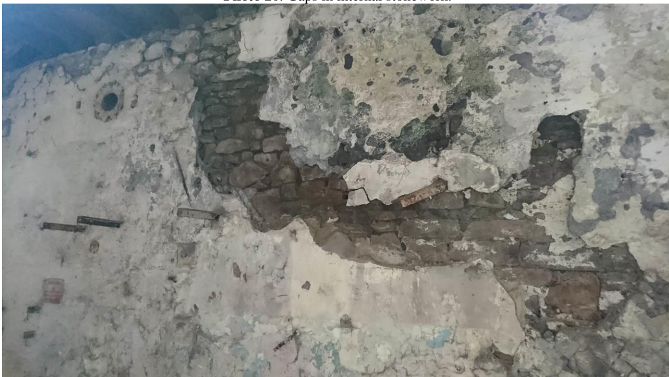
Photo 20: Gaps in internal stonework.
