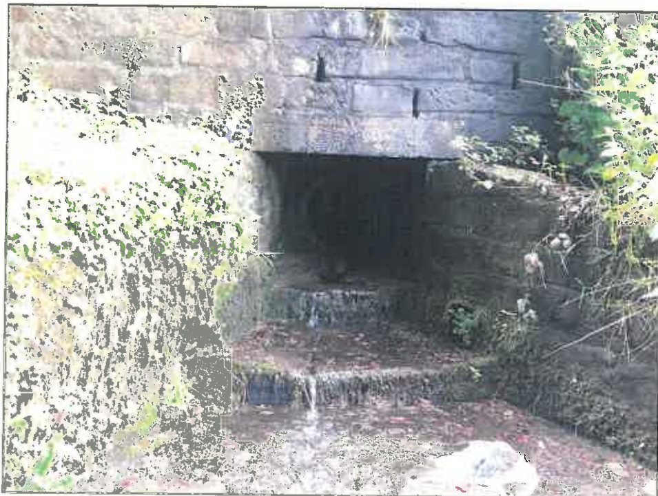
Plate 12: Culvert to north of site
