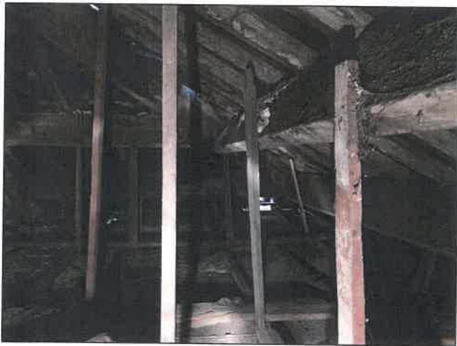
Plate 8: Roof void, west aspect
