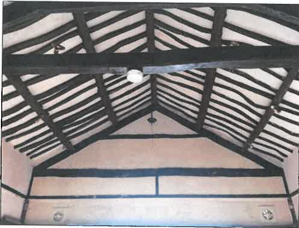
Plate 7: Mezzanine to northeast
