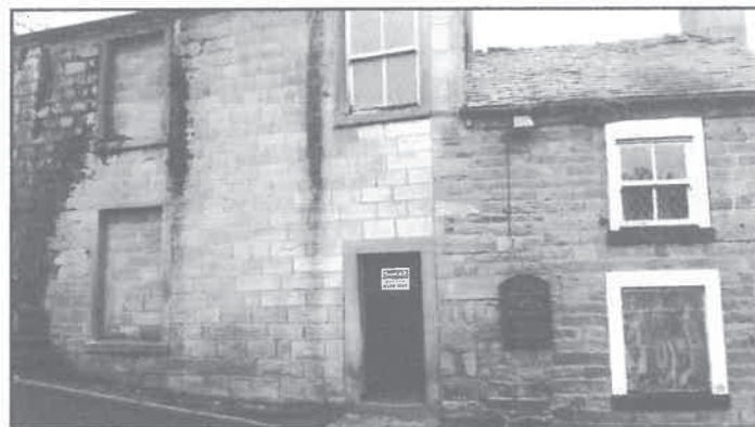
Figure 5) Eastern cottage (shown here to the right) with blocked door (behind notice board) and left hand later C19th addition (dwelling) at the eastern end of the building.
