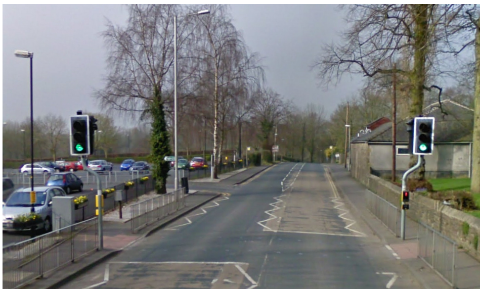
Figure 3.1 – Controlled Pedestrian Crossing on Edisford Road
