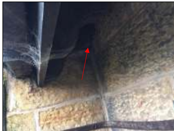
6a and 6b: Access point into roof underneath soffit at join between main church building and kitchen area, above the south-east corner of the flat roof behind the choir vestry
