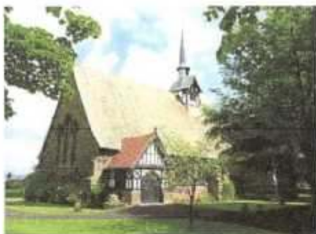
Figure 1: west and south elevations
