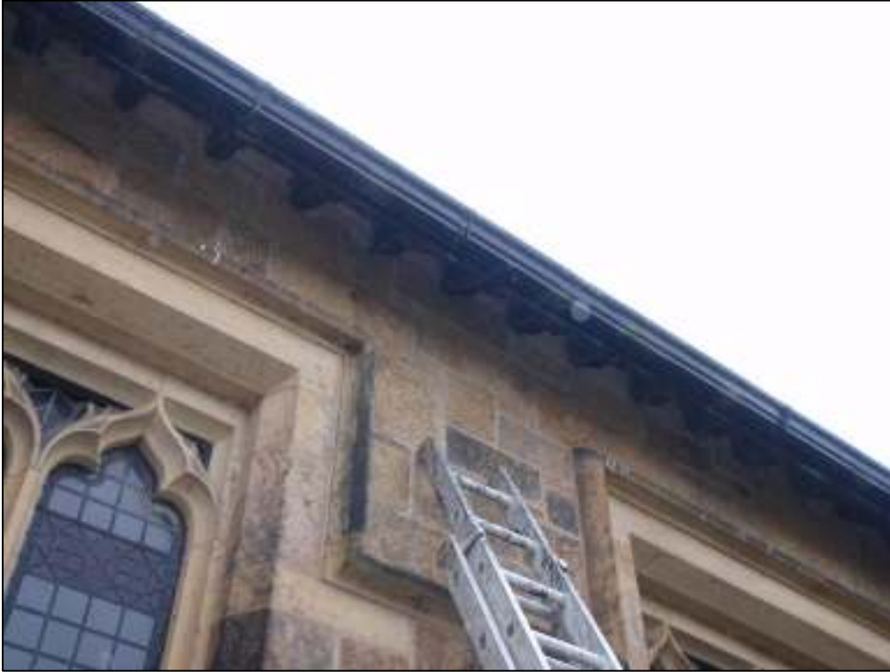
2a: North wall above second window (counting from the north-west corner of the church), showing the protruding rafter ends abutting the guttering
