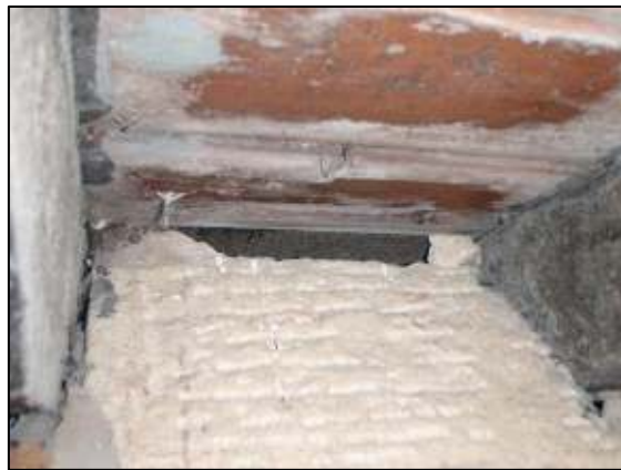
2b and 2c: Examples of gaps at top of north wall around second window, where mortar between the upper stones and the soffit and protruding ends of rafters has fallen out, giving access to a cavity
