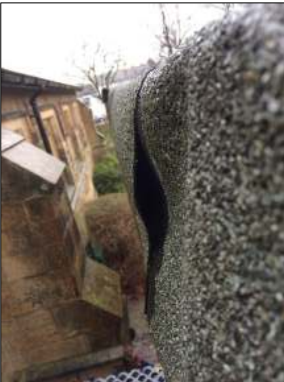
4a: Flat roof on choir vestry with roofing felt lifting, providing cavities in several places along this face
