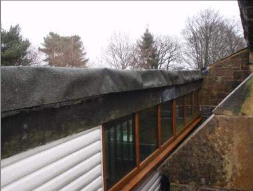
4a: Flat roof on choir vestry with roofing felt lifting, providing cavities in several places along this face
