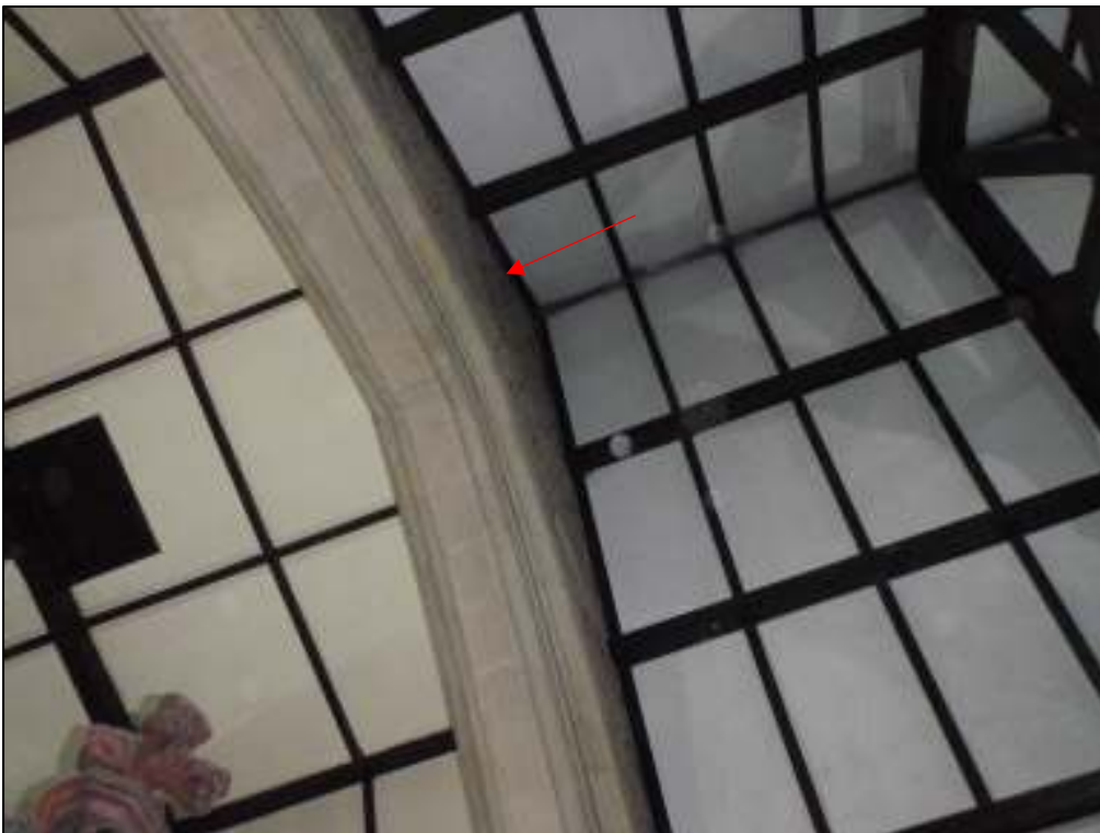
25: At the junction between the choir stalls and the nave, it was noted that the timbers on the roof above the choir stalls were not sat flush with the stone arch, creating a possible roost space. This was too high to examine, but based on the condition of the church interior, access into the roof space is unlikely
