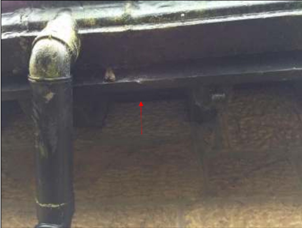
3a: 3.5 cm wide gap at join between wall and soffit, under main roof opposite choir vestry. Evidence of use by roosting birds (droppings visible in photograph)
