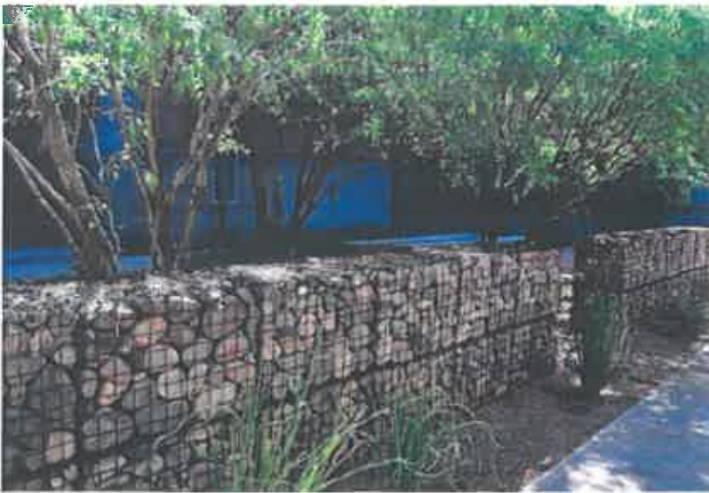
Example of Gabion retaining wall
