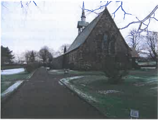
West elevation (from Lovely Hall Lane)
