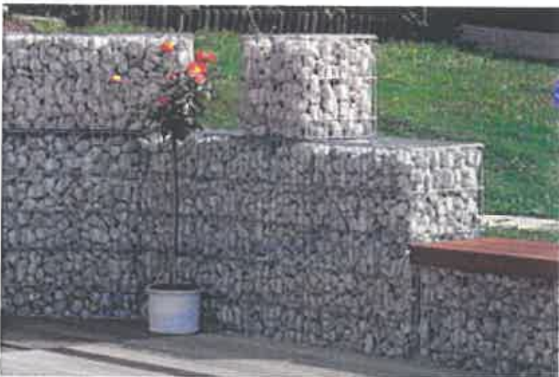
Example of Gabion retaining wall
