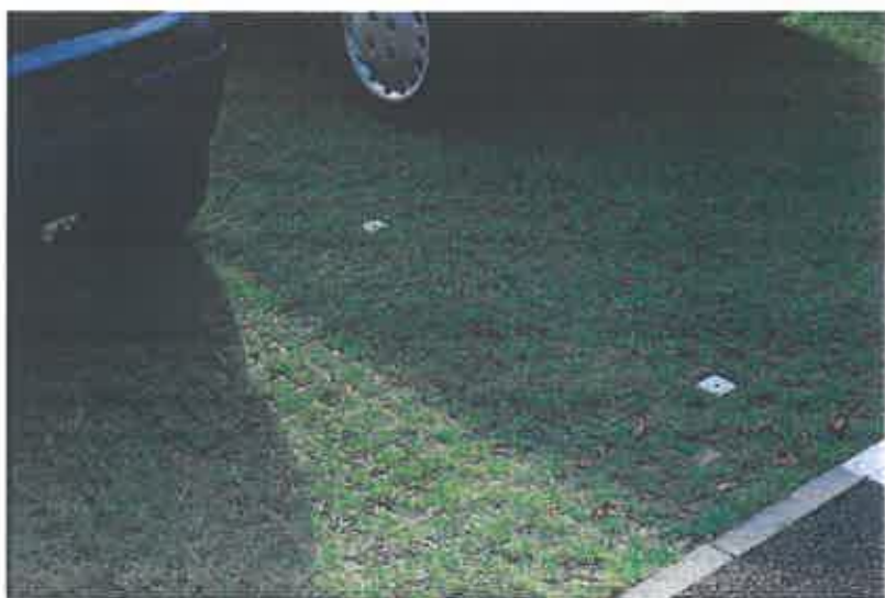
Geo-grid grass reinforcement to the car park
