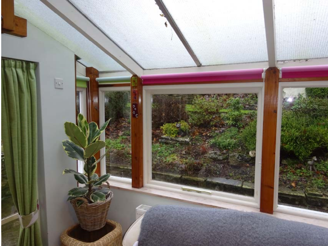
Timber posts supporting rafters, timber casement windows
