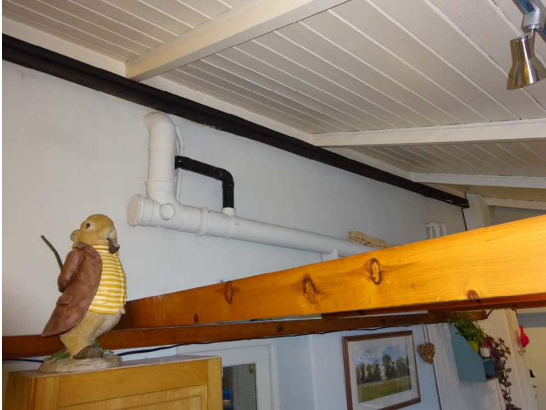
Mono pitched roof - close boarded timber below slates supported by timber rafters
