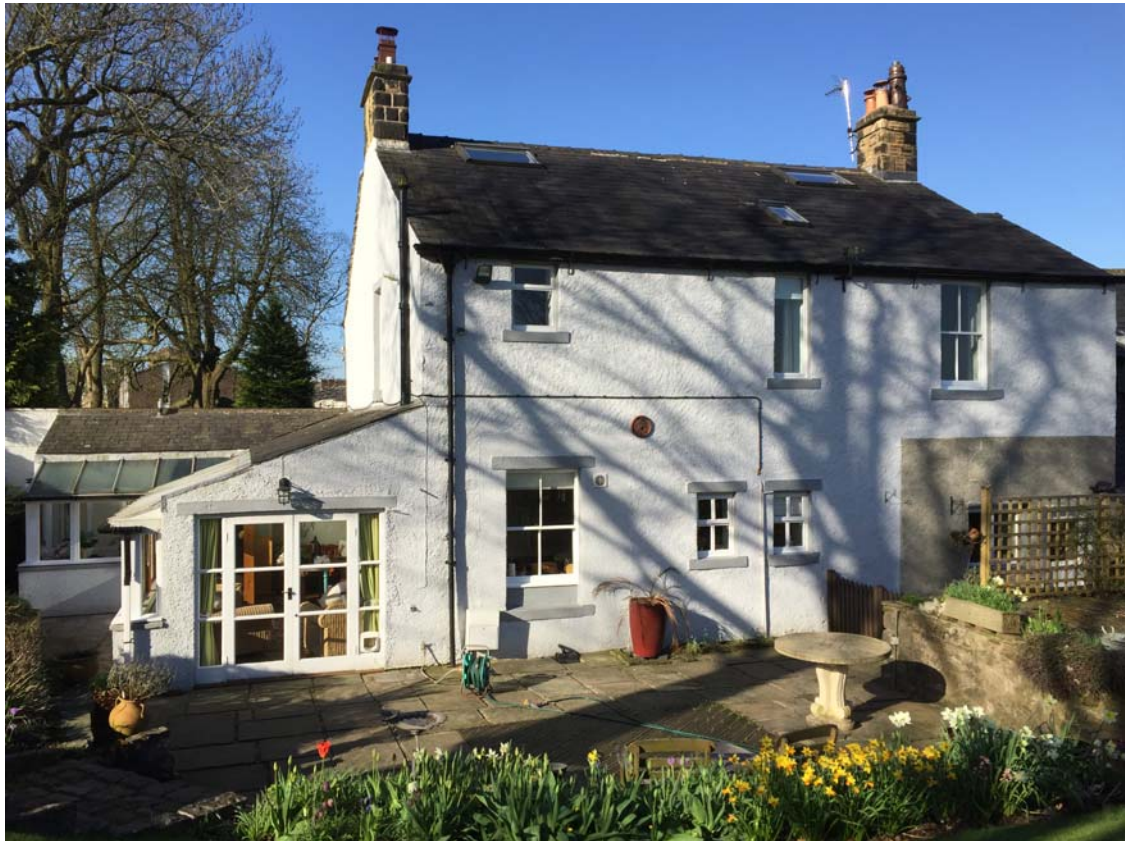
Ashgrove House / Side Addition – Rear Elevation
