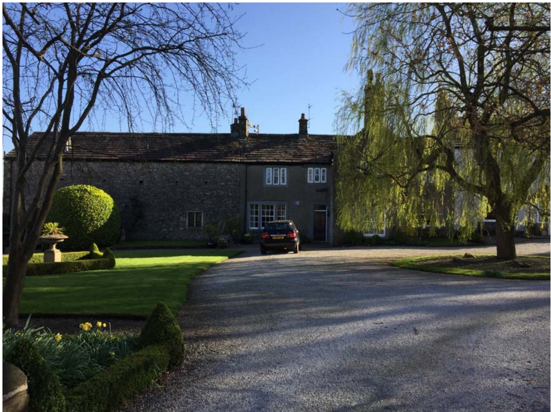
Ashgrove Barn/ Shaw Cottage – Front Elevation
