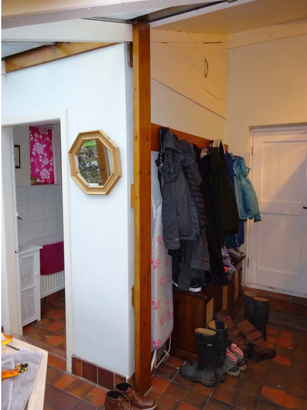
Internal blockwork wall, quarry tiled floor and skirtings
