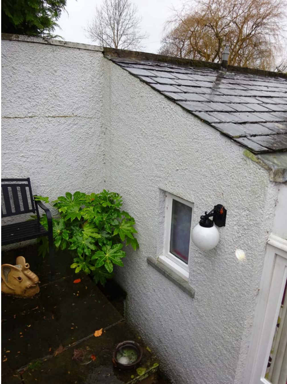
Front Boundary Wall – Cement render over concrete blockwork cavity wall and topped with stone copings, painted timber casement window and pre-cast concrete sill
