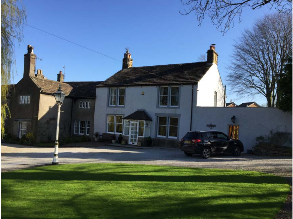
Shaw Cottage / Ashgrove House – Front Elevation
