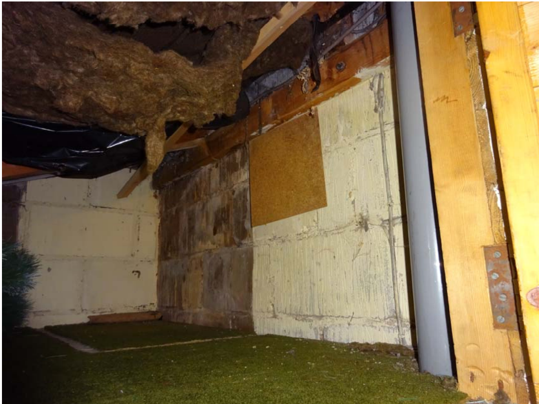
Storage space above WC - blockwork cavity walls to front boundary and side elevation
