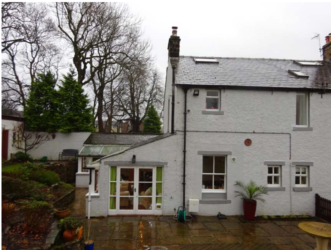
Rear Elevation – Main Building & Single Storey 1970's Lean-to Addition
