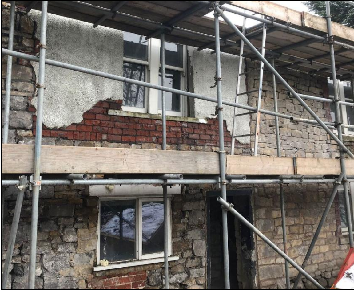
Figure 5) Rear elevation during render removal showing full height joint right of doorway and partial brick walling at first floor and beneath the ground floor window.
