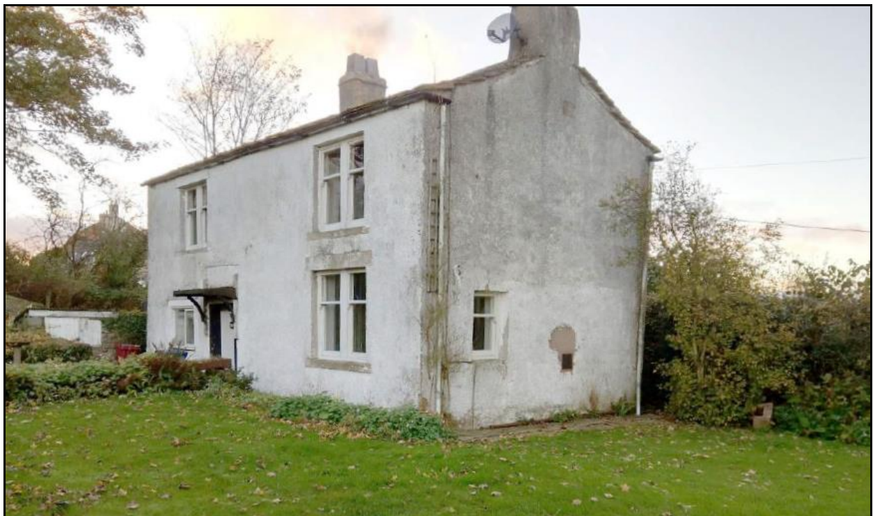
Figure 4) Rear (southern) elevation prior to removal of render
