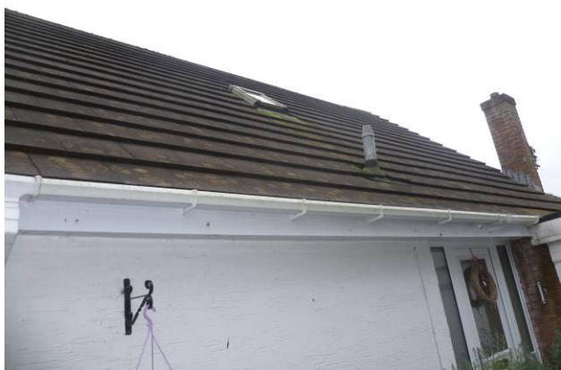
NW side elevation, concrete tiles are tight fitting with no gaps.
