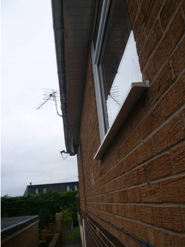
SE side elevation with tight fitting soffits.
