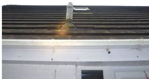
NW side elevation, concrete tiles are tight fitting with no gaps.
