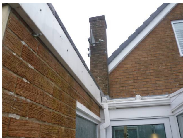
SW rear elevation (part) and side of garage with tight fitting fascia boards (no gaps)
