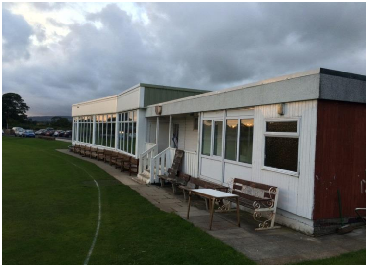
Plate 3.1 showing the exterior construction of the cricket pavilion
