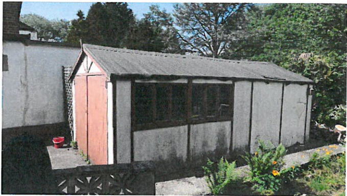
Figure 8: an old garage / shed at rear of property
