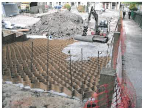
Appropriate aggregates are back filled filling all of the cells
