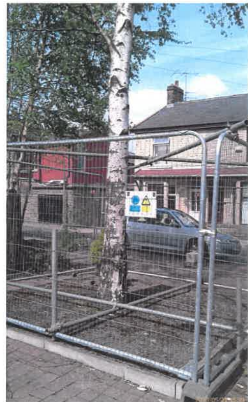
Site photos of protective fencing on site with warning / information sign fixed to the fencing
