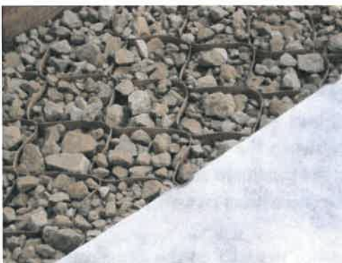
Geotextile fabric laid over filled cells then covered with temporary / permanent wearing course as per construction specifications
