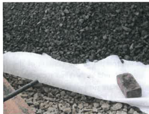
Geotextile fabric laid over filled cells then covered with temporary / permanent wearing course as per construction specifications
