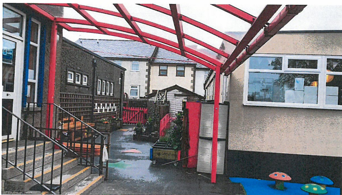
Existing Nursery Building – Gable End
