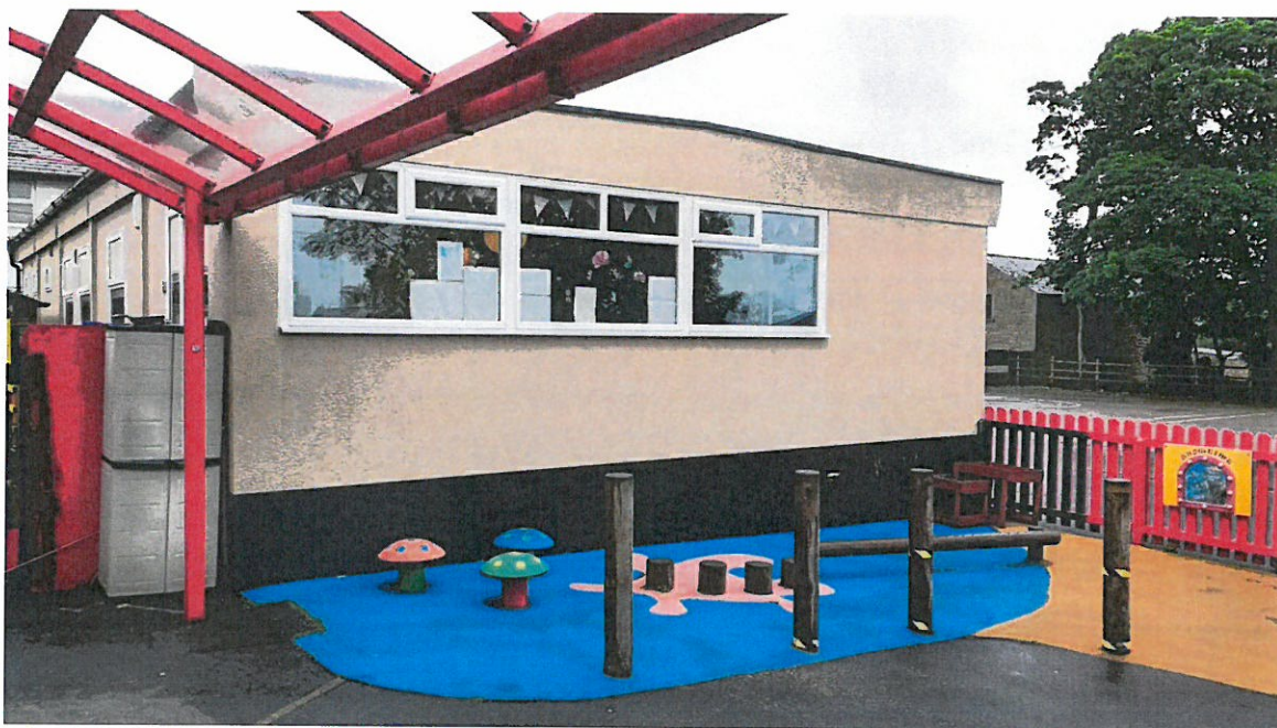
Existing Nursery Building – Gable End
