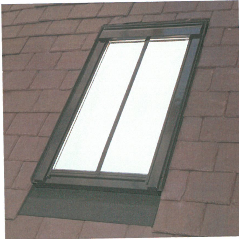
PL05: Indicative Image of recessed conservation roof light with central glazing bar.
