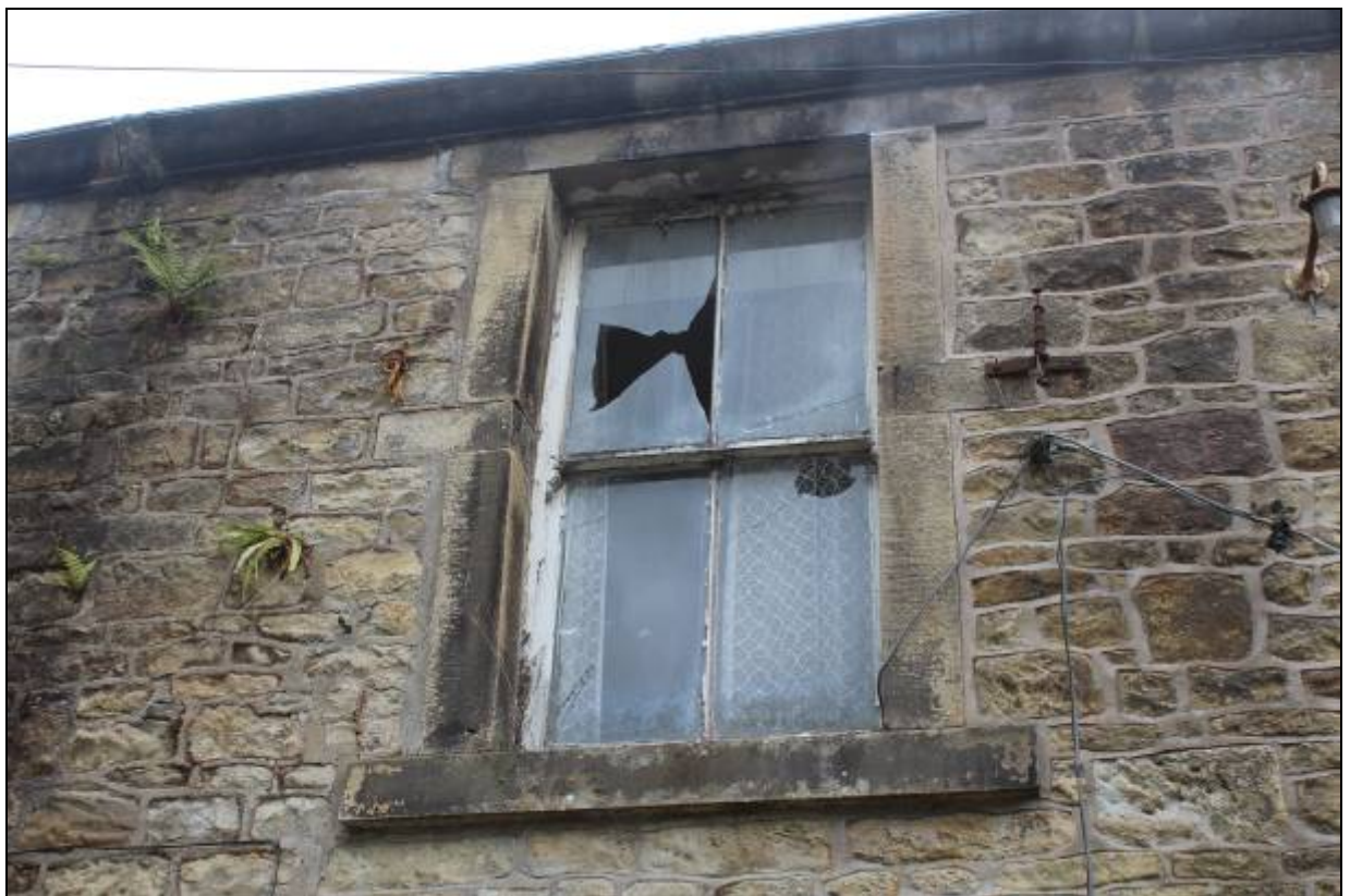
7. Windows are typical mid-later 19 th century four-paned horned sashes
