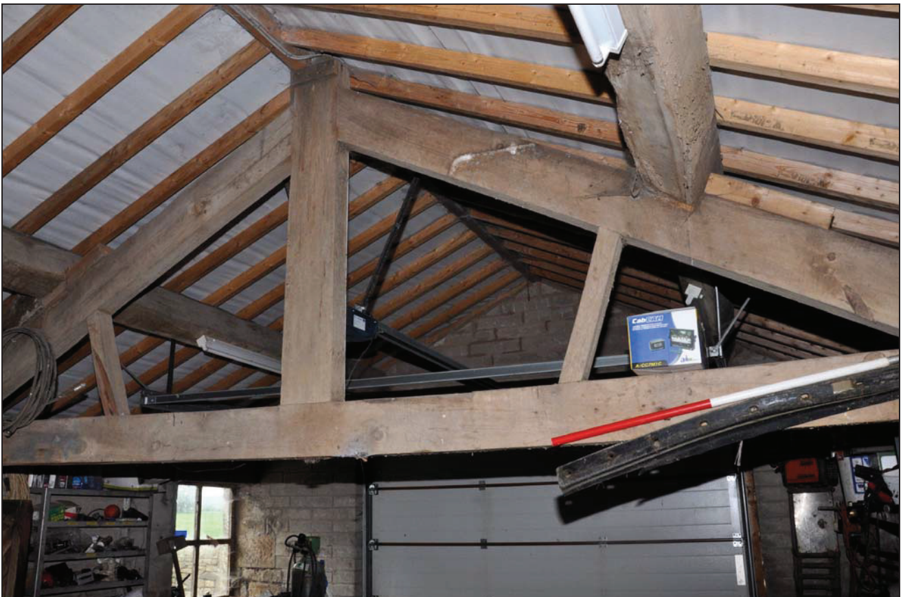
Photo 28: Former cart shed (building 3): roof truss
