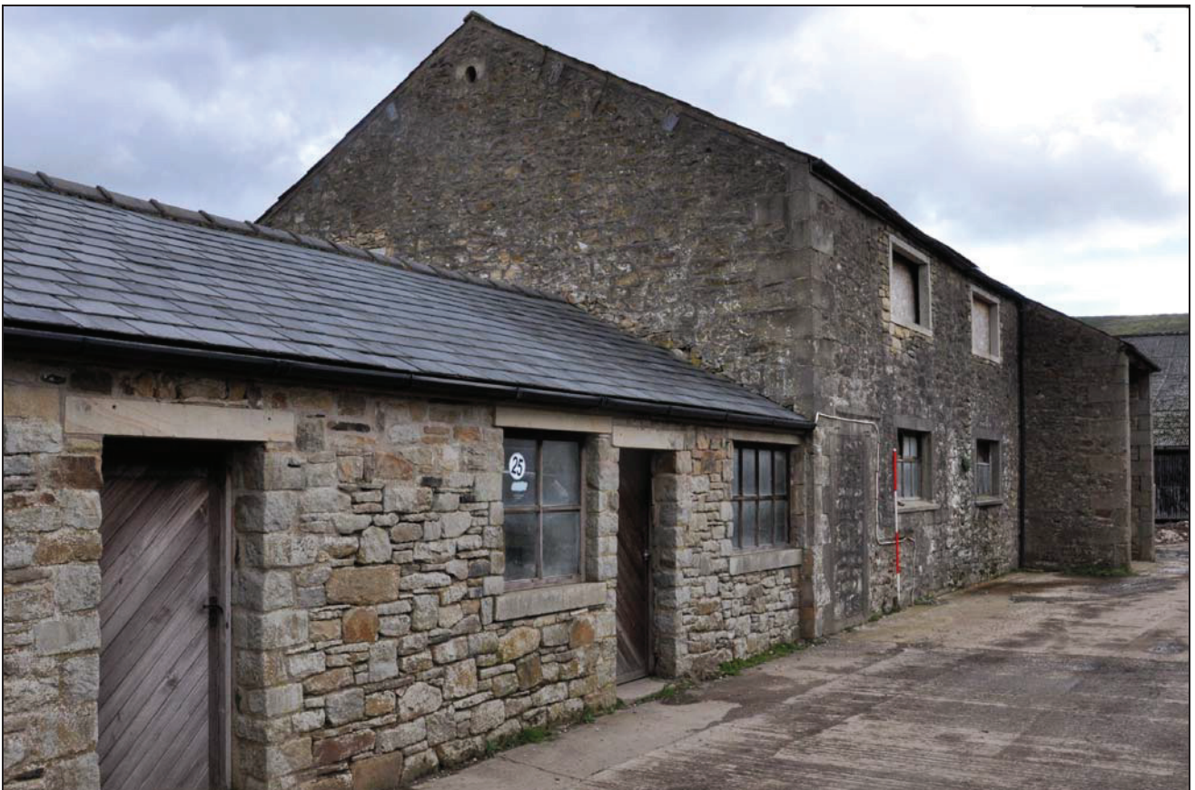
Photo 8: Barn (building 1): general view, looking east
