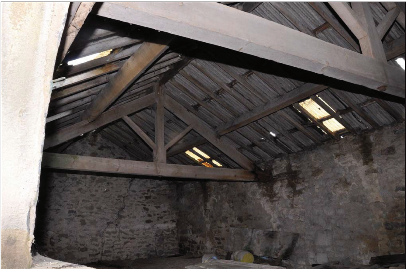
Photo 24: Former stables (building 2): first floor, looking west
