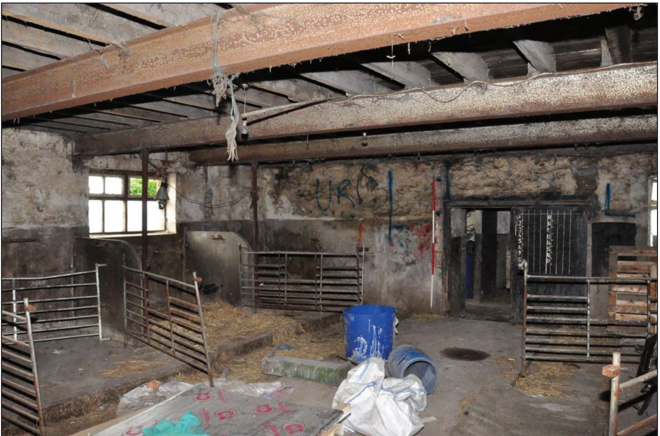
Photo 10: Barn (building 1): ground floor, looking west
