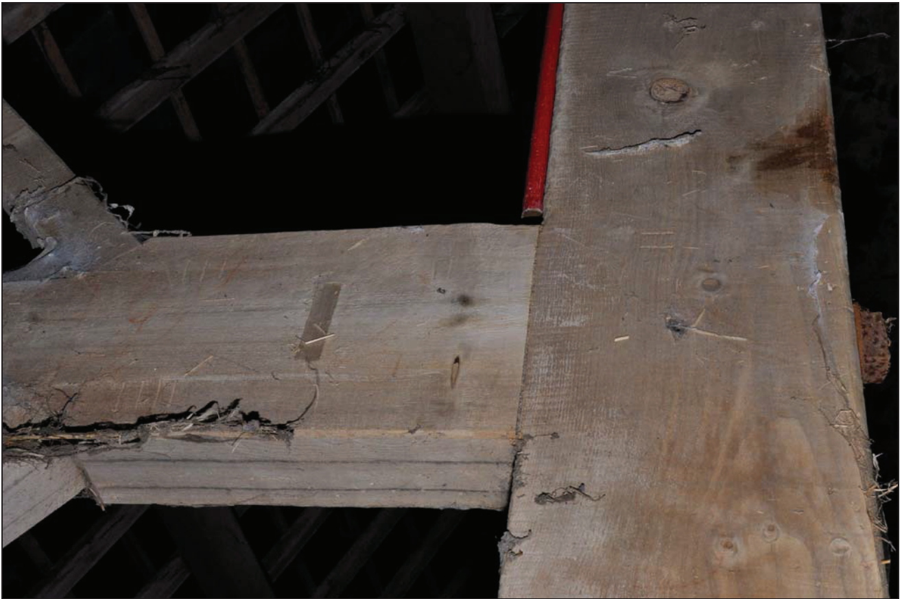
Photo 14: Barn (building 1): detail of carpenter's marks on central roof truss
