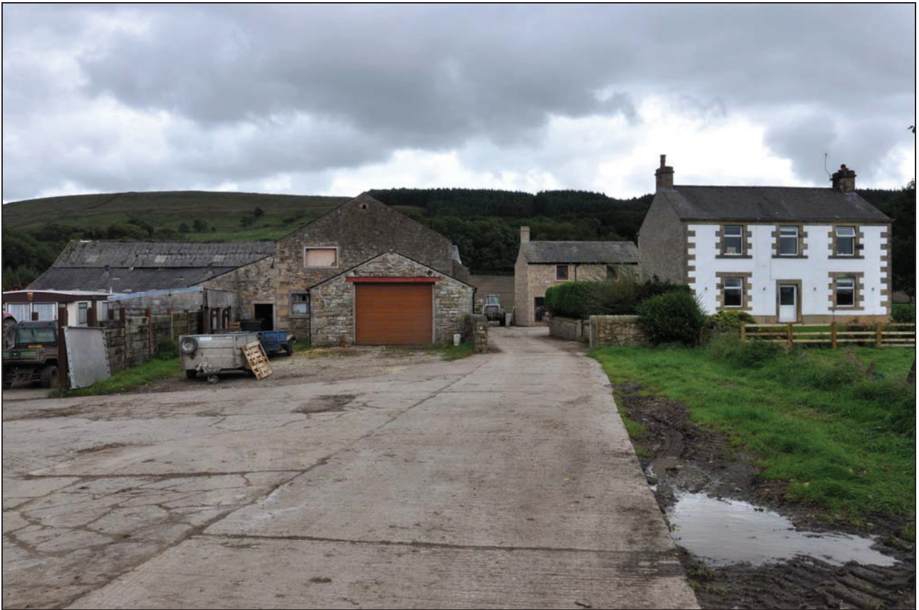
Photo 1: General view of the farmstead from the north-west, with buildings recorded to left
