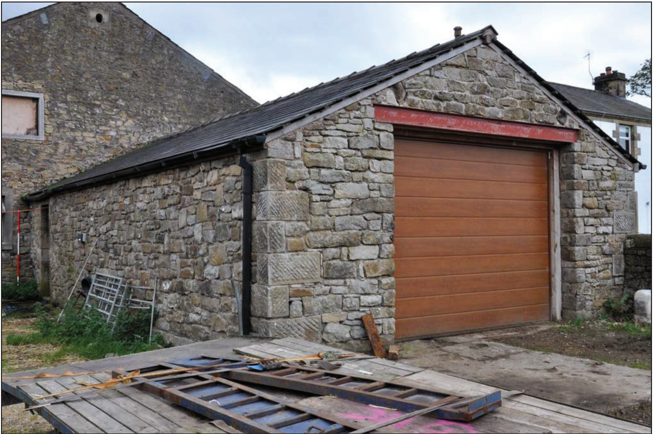
Photo 27: Former cart shed (building 3): general view, looking south
