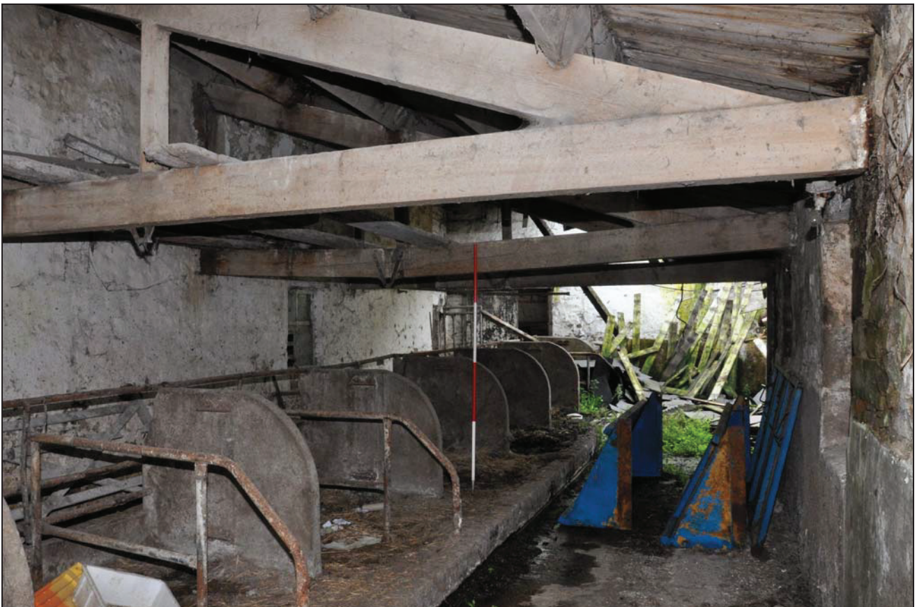
Photo 31: Lean-to shippon (building 4): interior, looking south-west
