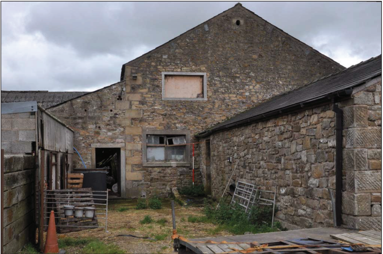
Photo 9: Barn (building 1) and shippon (building 4): north-west elevations
