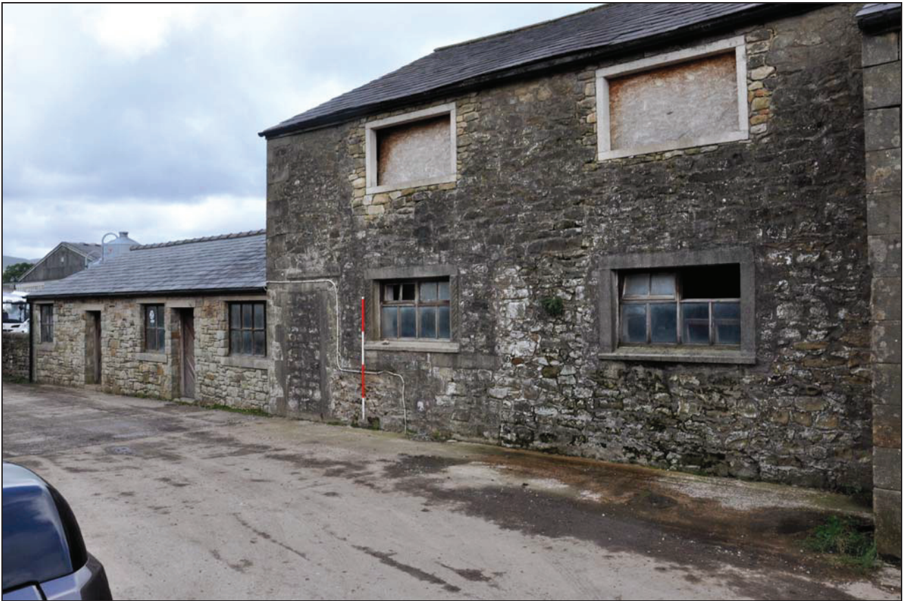
Photo 3: Barn (building 1) and former cart shed (building 3): south-west elevations
