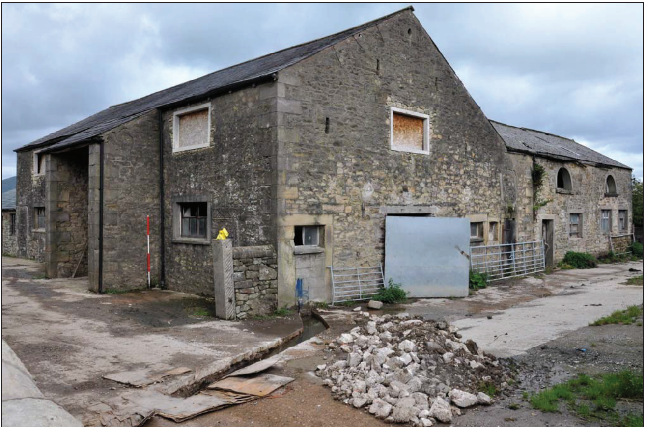
Photo 4: Barn (building 1) and former stables (building 2): south-east elevations
