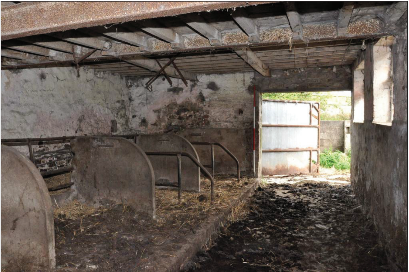
Photo 23: Former stables (building 2): ground floor, looking north-east
