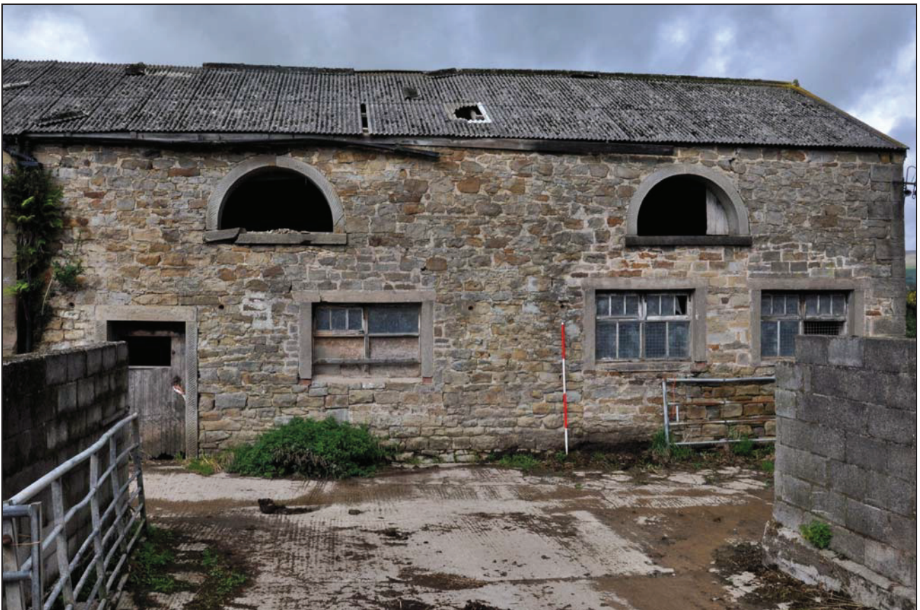
Photo 16: Former stables (building 2): south-east elevation
