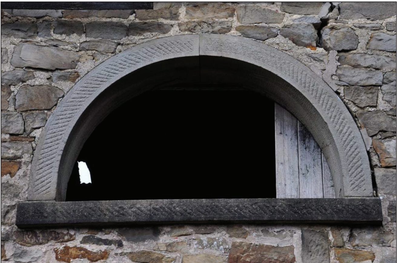
Photo 20: Former stables (building 2): detail of forking hole, south-east elevation
