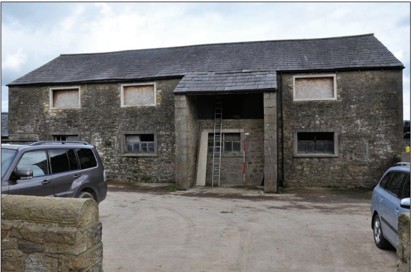
Photo 2: Barn (building 1): south-west elevation
