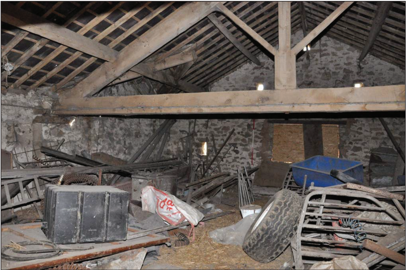
Photo 12: Barn (building 1): first floor, looking east
