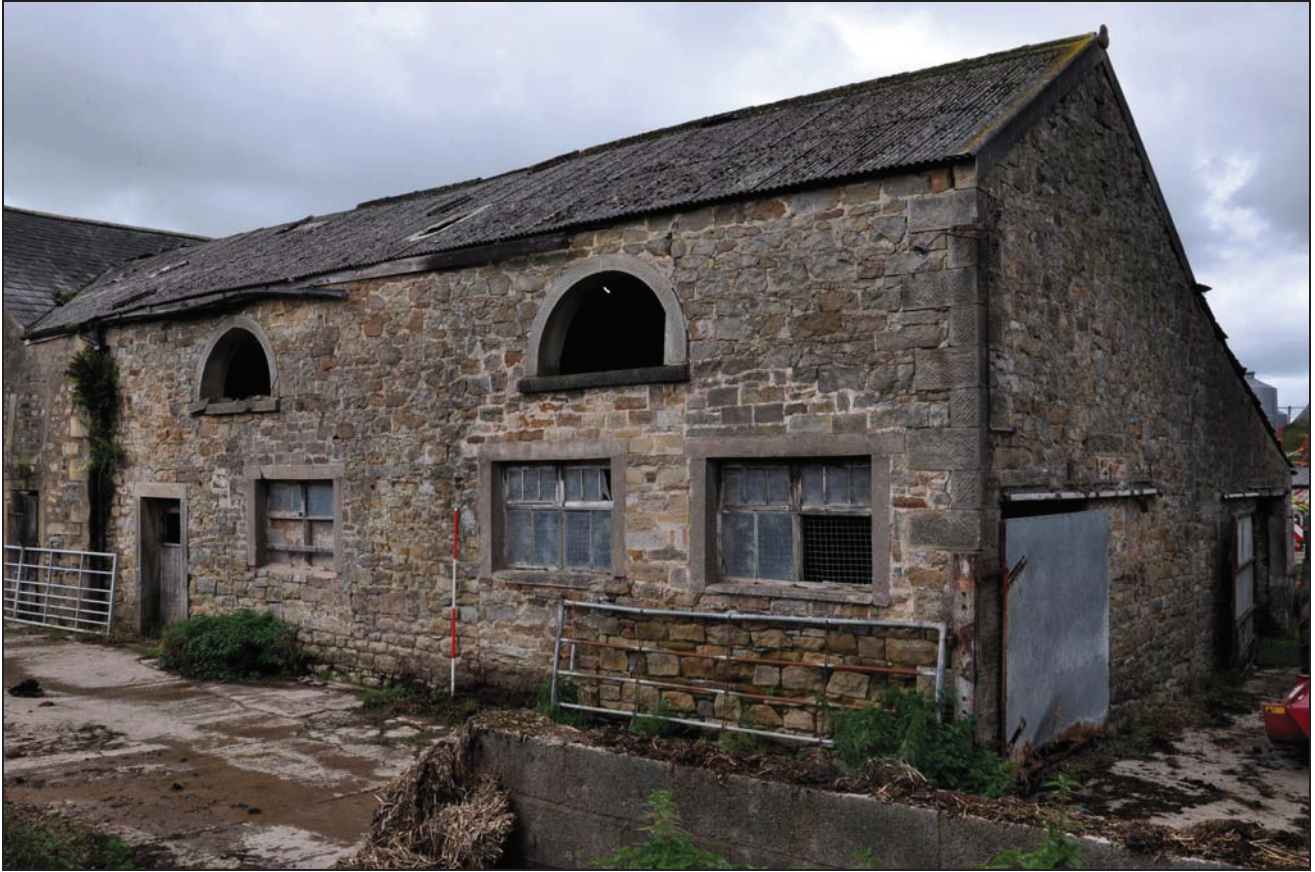
Photo 19: Former stables (building 2): south-east elevation
