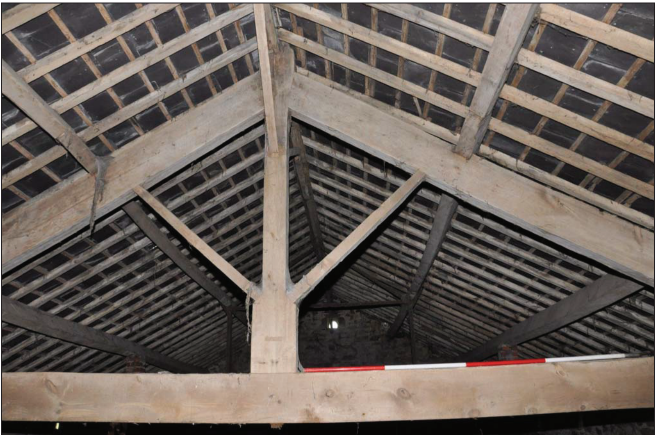
Photo 13: Barn (building 1): central roof truss, looking north-west
