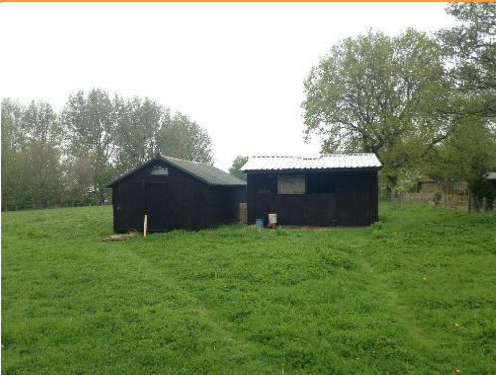
PLATE 7 – TWO SHEDS IN THE EASTERN SECTOR OF THE SITE
