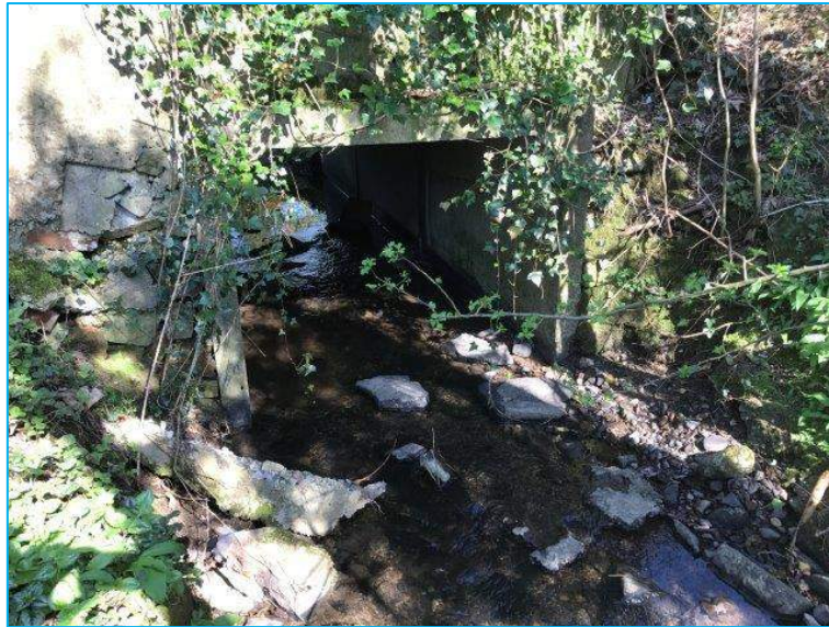
Figure 7 - Culvert on the Drainage Ditch
