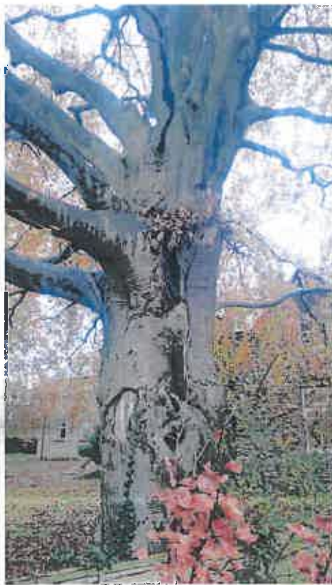
Tree T2; note tears at 2 and 5 metres
