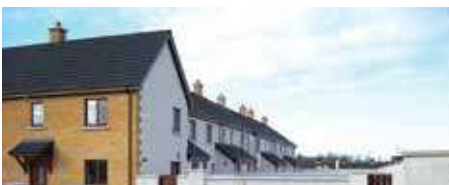
Social Housing Installation Co. Louth, Ireland
