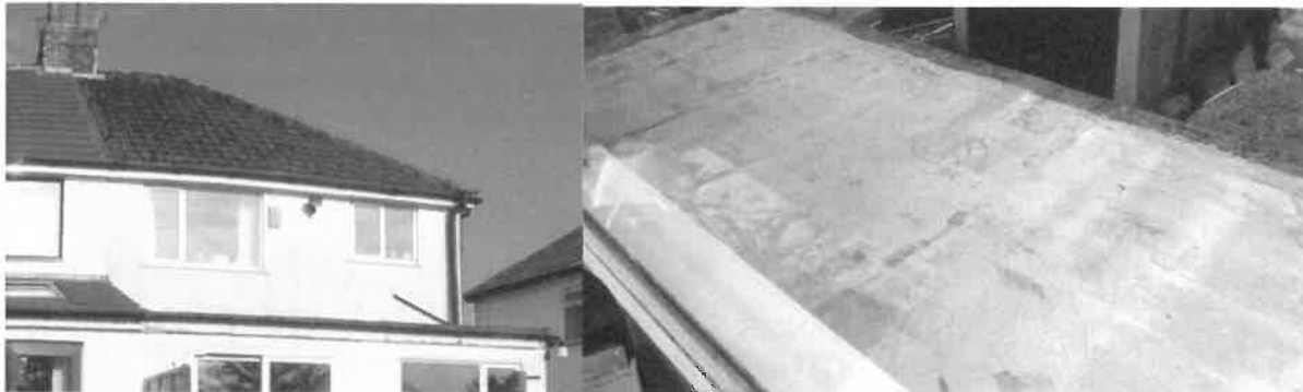
Flat roof finish
