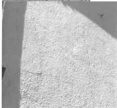
The walls are white painted render, with a brick plinth.
