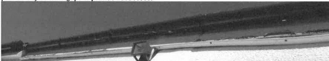
Flat roof fascias
