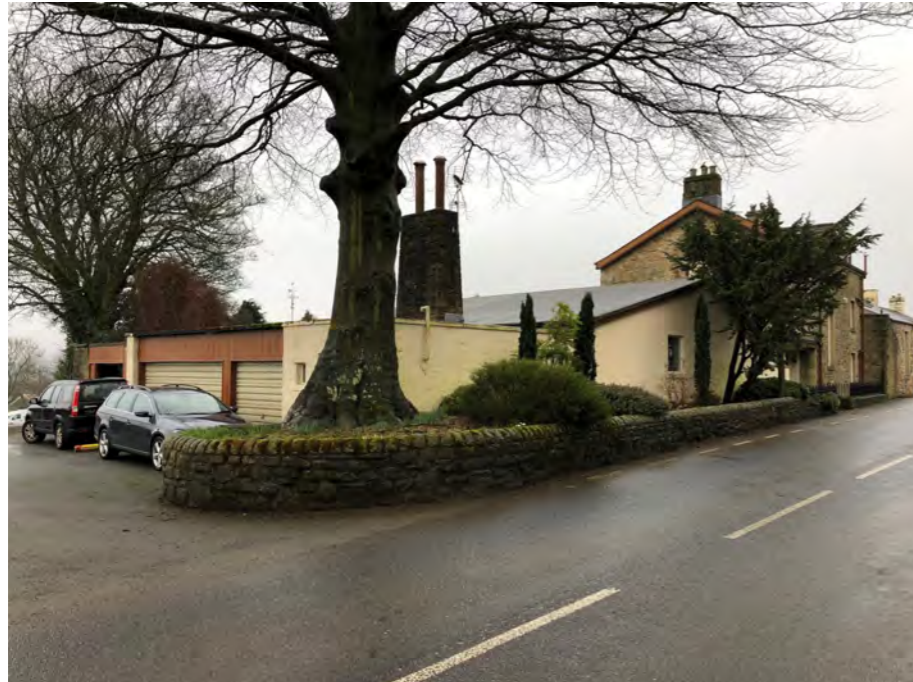
External view of Prospect House from across the street. Shared access past garages (left) to farm, music room, hallway and original house (right).
