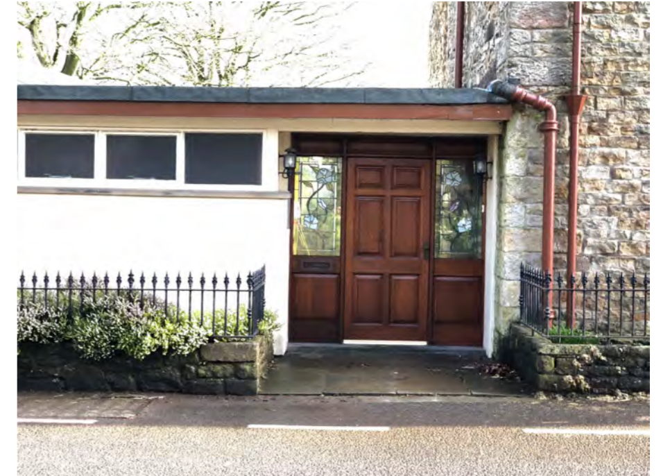
Front access directly from road with no protection
