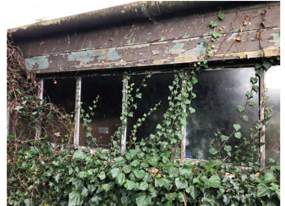
External view of rear part of garage
