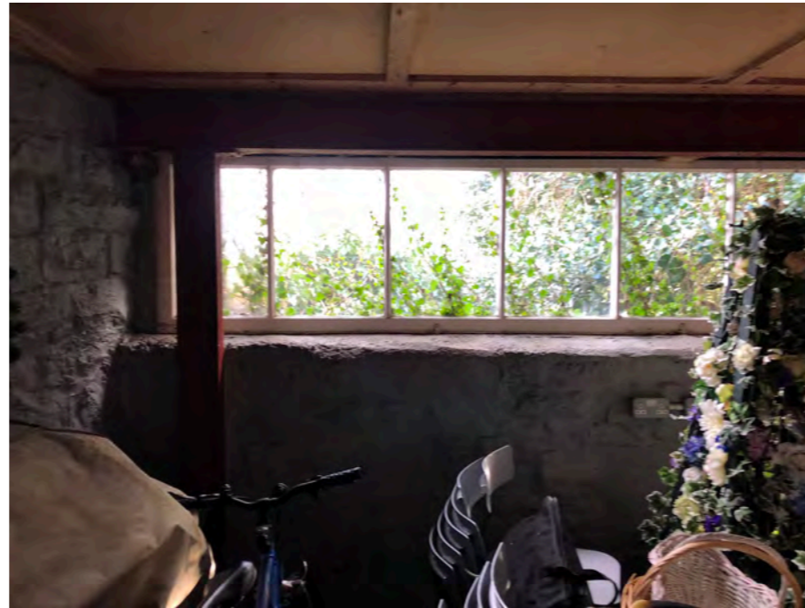
Internal view of rear section of garage
