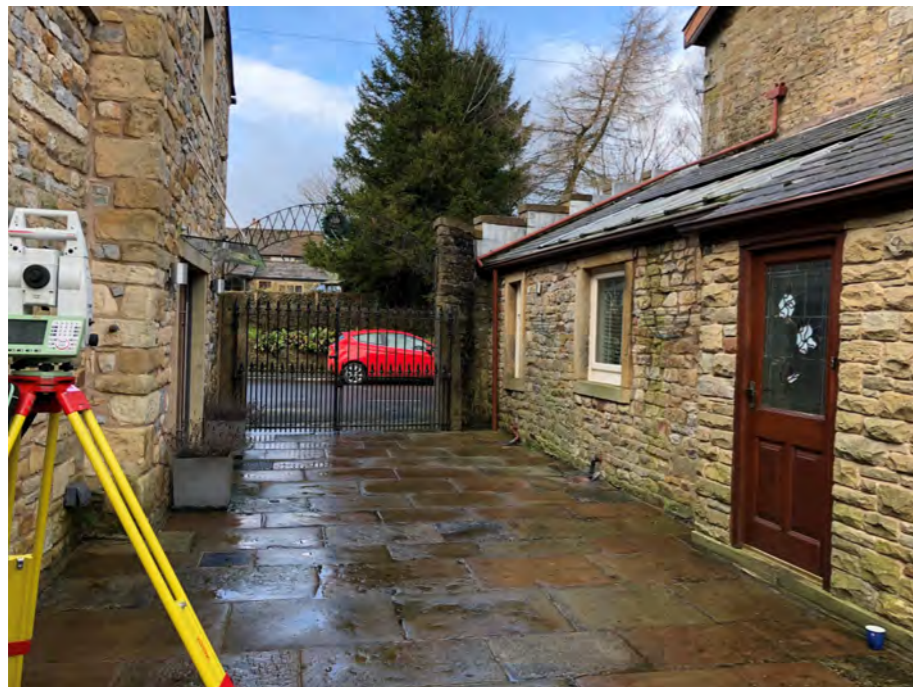
Courtyard access and parapet wall along side lean-to
