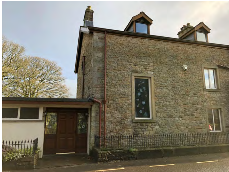
Roadside elevation, including more modern additions of dormers and hallway link to music room.
