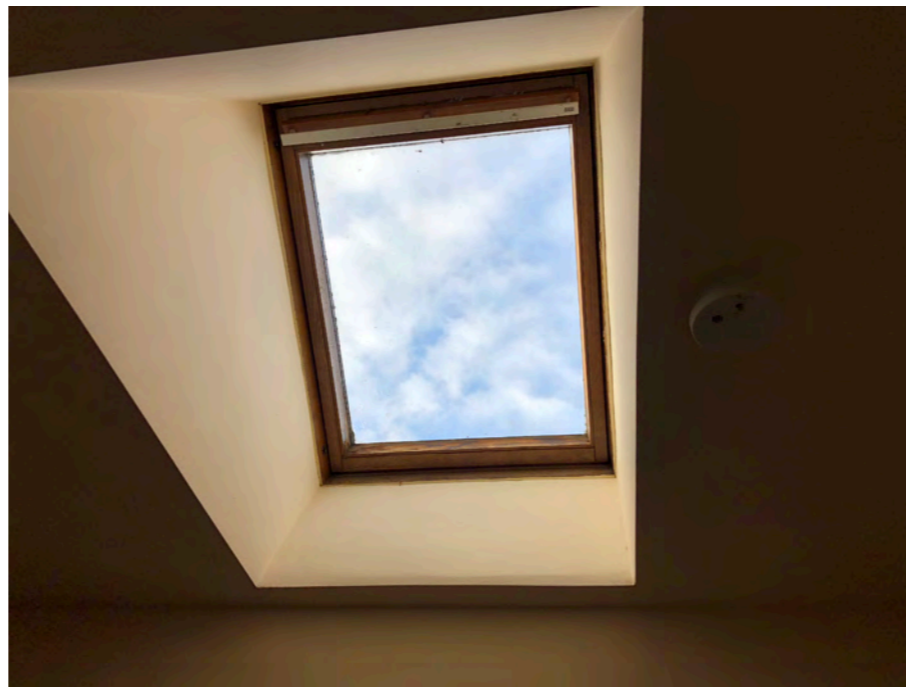
Internal view of roof light
