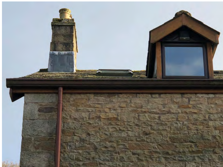
External view of dormers
