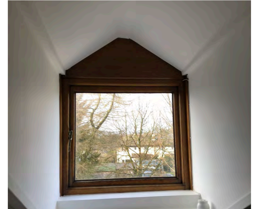
Internal view of dormers
