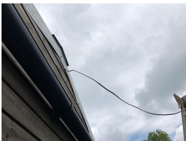
Photo 21: Gable end with lifted flashing
