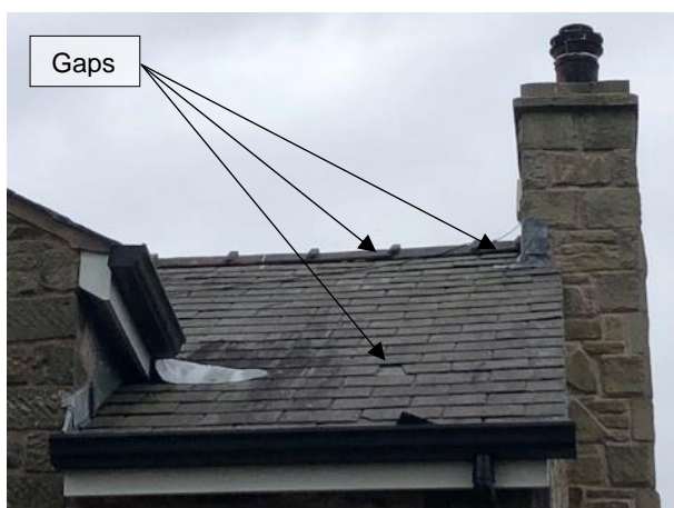
Photo 2: Example locations of gaps beneath roof tiles
