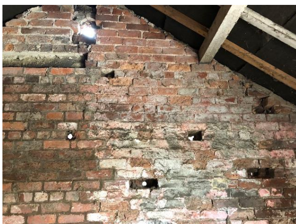
Photo 16: Gaps within south-eastern gable wall
