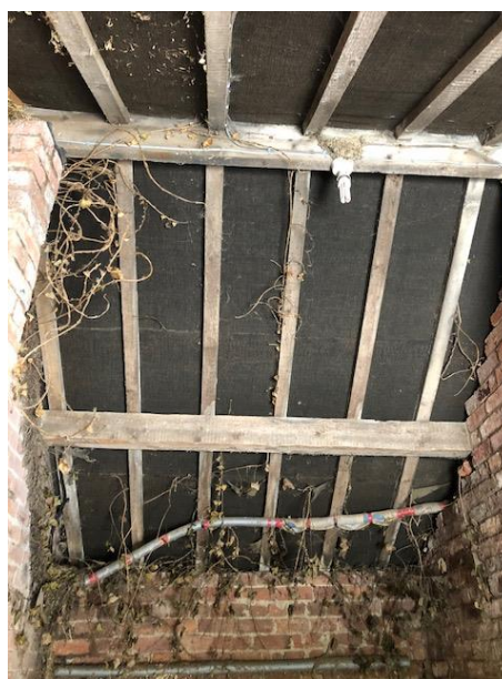
Photo 18: Felt sarking and ivy growth
