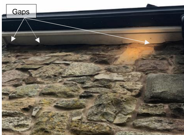
Photo 3: Typical gaps along soffit boxes at eaves
