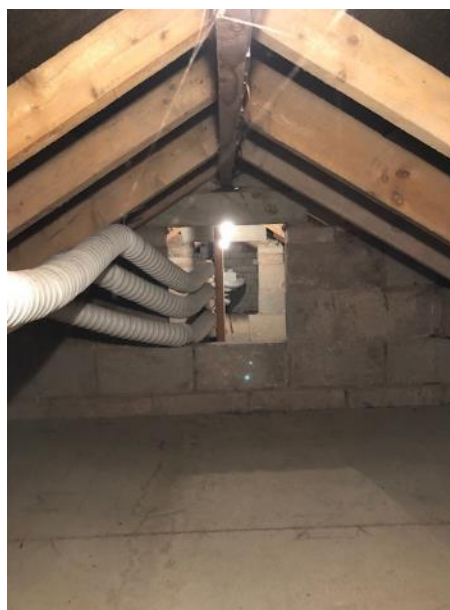
Photo 8: Breezeblock supporting walls of Loft Space C – looking north-east
