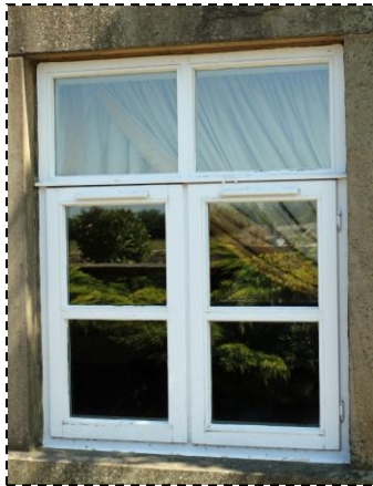
Fig 3 - Existing double glazed timber side hung casements & fixed light windows
