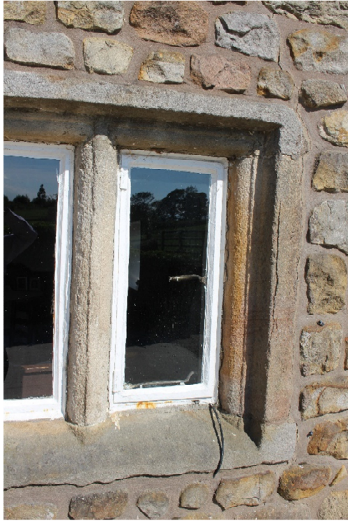
Photo No.7 Front window detail
