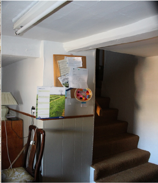
Photo No.8 Internal wall originally the rear wall & staircase
