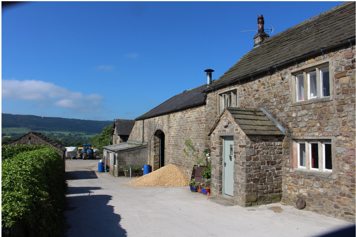
Photograph N0.1 Masons Farmhouse & Barn. Grade II Listed Building
