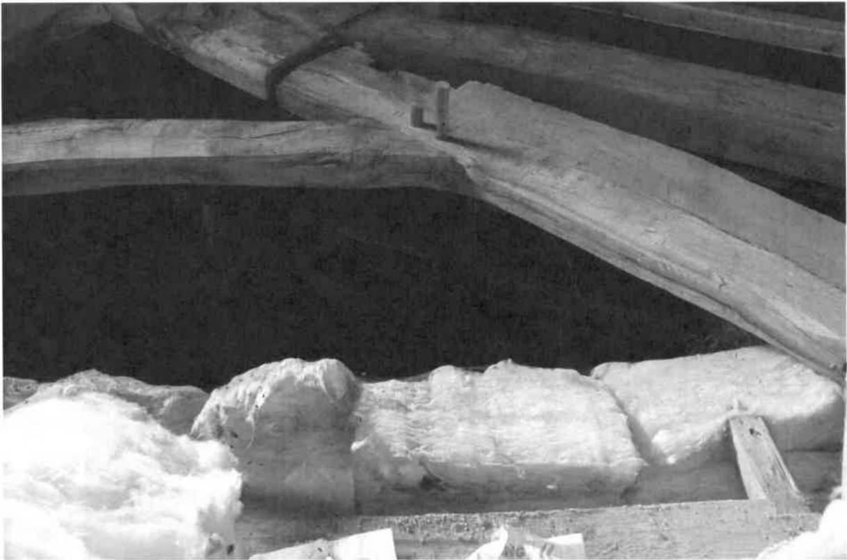
Photo of the altered roof truss.
