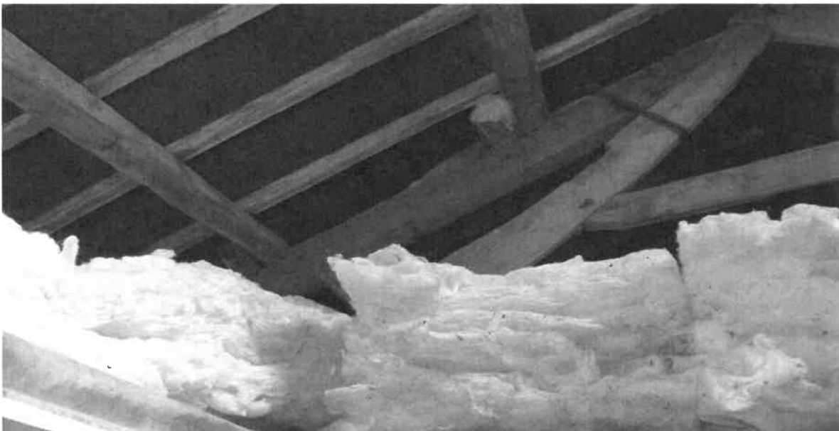
Photo showing added top chord and purlins
