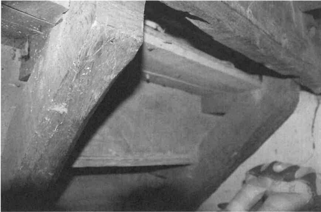
This photo shows the present staircase supported on a similar timber.
