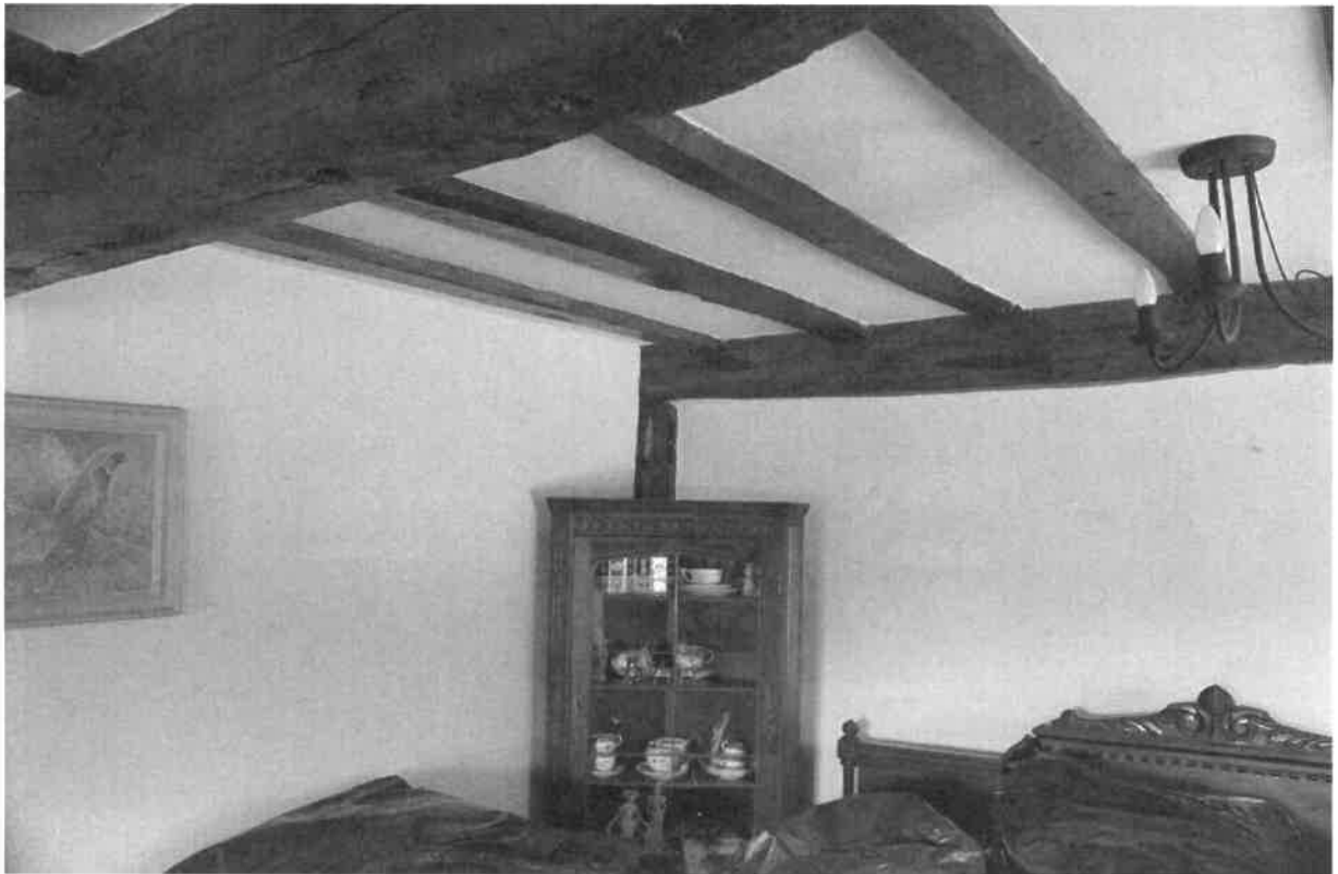
Ceiling in the front right- hand room showing ceiling and beam end with post support
