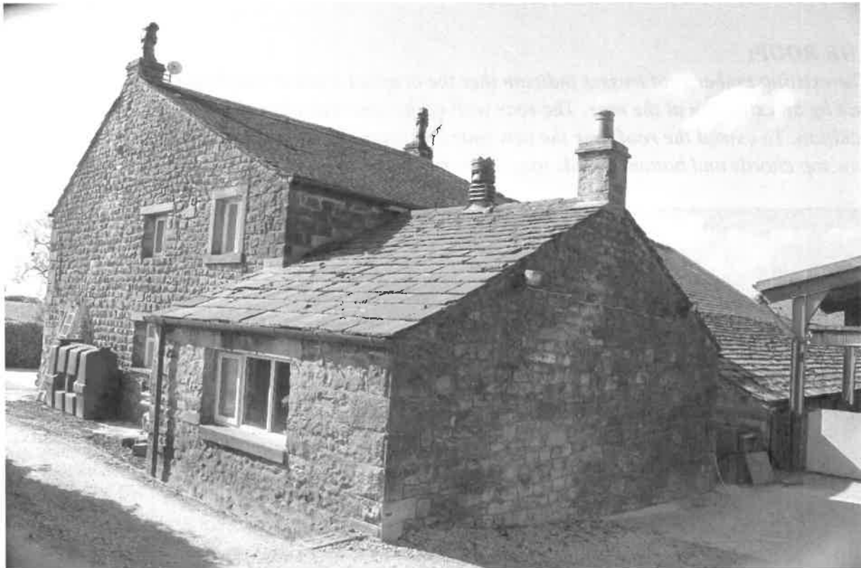
This photo shows a later second single storey extension
