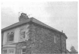
The property consists of a brick built semi detached two storey house with multi pitch slate roof. The first floor front wall and rear ground floor is rendered. A single storey single pitch roofed extension is present to the rear. Roofs feature well sealed ridge tiles and close fitting slates. Lead flashing is in good condition and close fitting.
