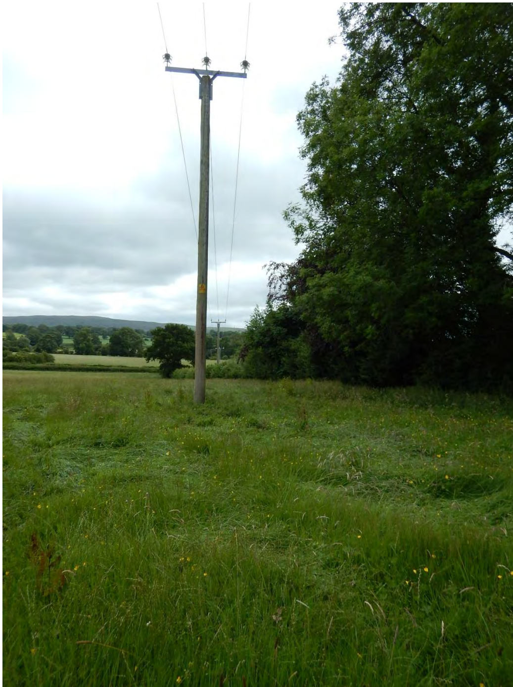
Photograph 5: Southernmost utility poles on western side
