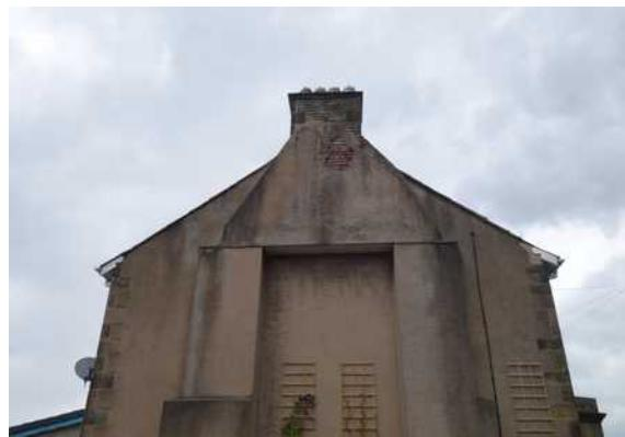
The property consists of a stone built two storey end terrace with partially rendered external walls. The building has a double pitched slate roof in a good state of repair with a well sealed ridge. Lead flashing is close fitting with no noticeable gaps or crevices.
