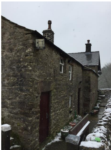
Photos illustrating the outer skin of stonework which requires stabilisation works.
