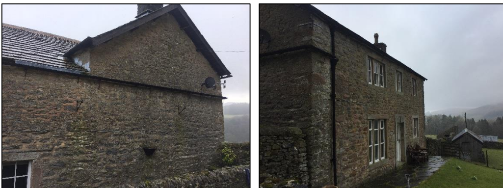
Plates 1 and 2: Southern and eastern elevations of farmhouse.
