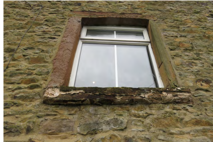
Ground floor rear window
