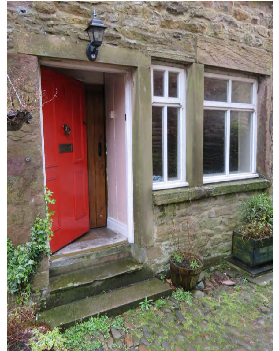
Front elevation and main access door
