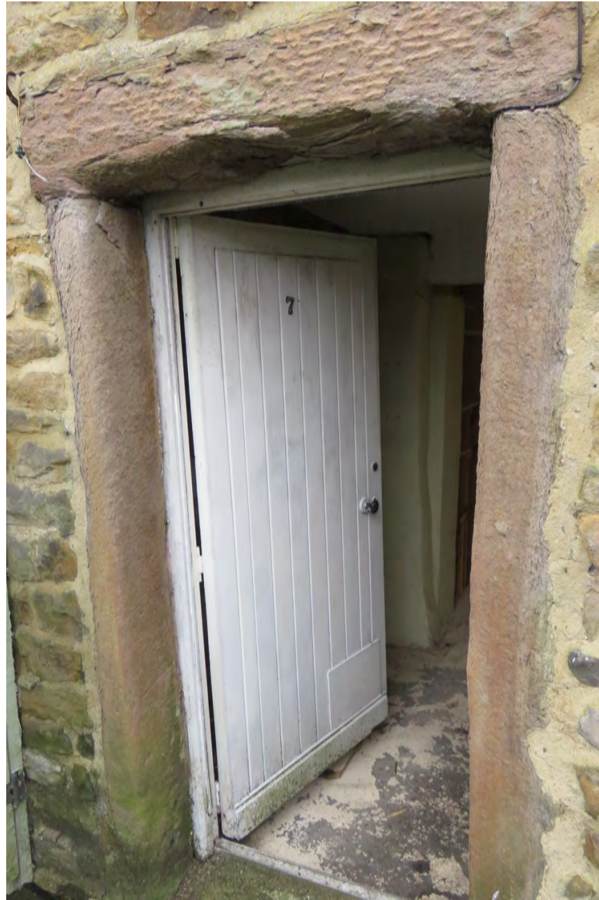
Lower ground floor, access to yard
