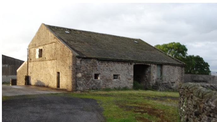
Figure 1: Stone barn at Witton's Farm (NE elevation)
