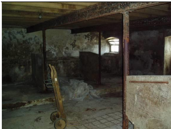
Shippon with hay loft on metal columns
