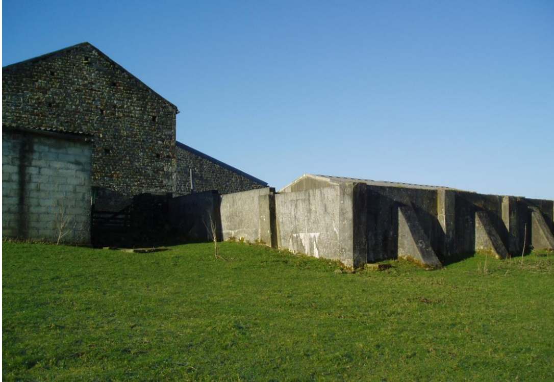
4 Concrete area with surrounding retaining walls are being demolished.
