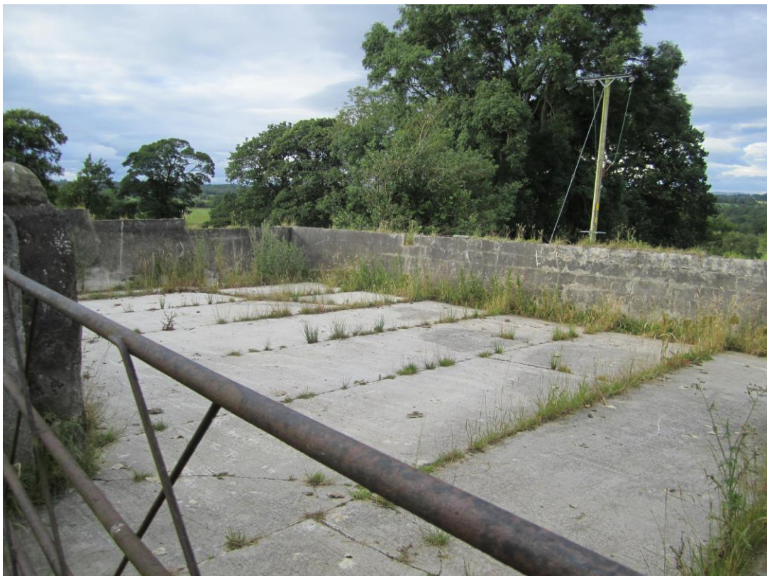
3 Concrete area with surrounding retaining walls which are being demolished.
