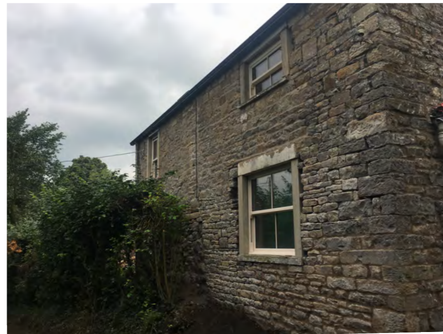
View of cottage from road side
