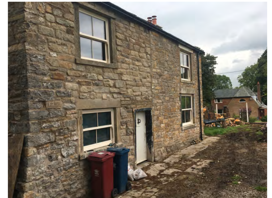
Rear elevation with front door
