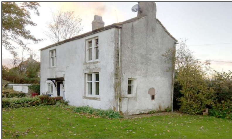
Figure 7) Rear (southern) elevation prior to removal of render
