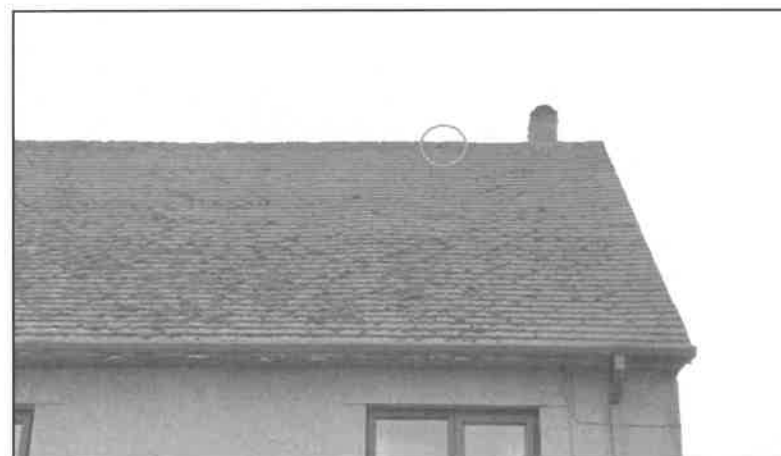
Photo 7: Broken ridge tile
