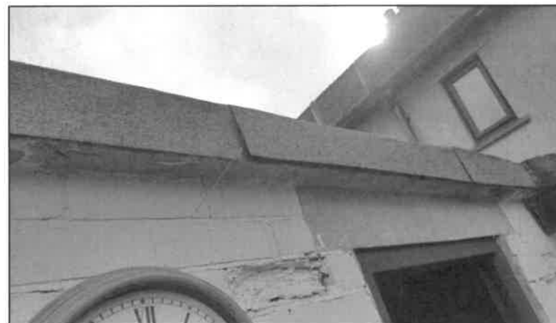
Photo 6: Gap in overlap fold of felt roof of flat roof section – arrow indicated where it is open at one side.
