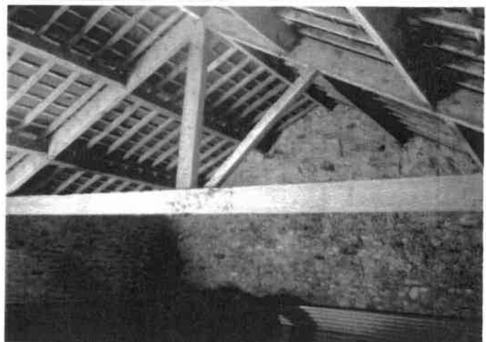
18. Roof with King Post trusses.
