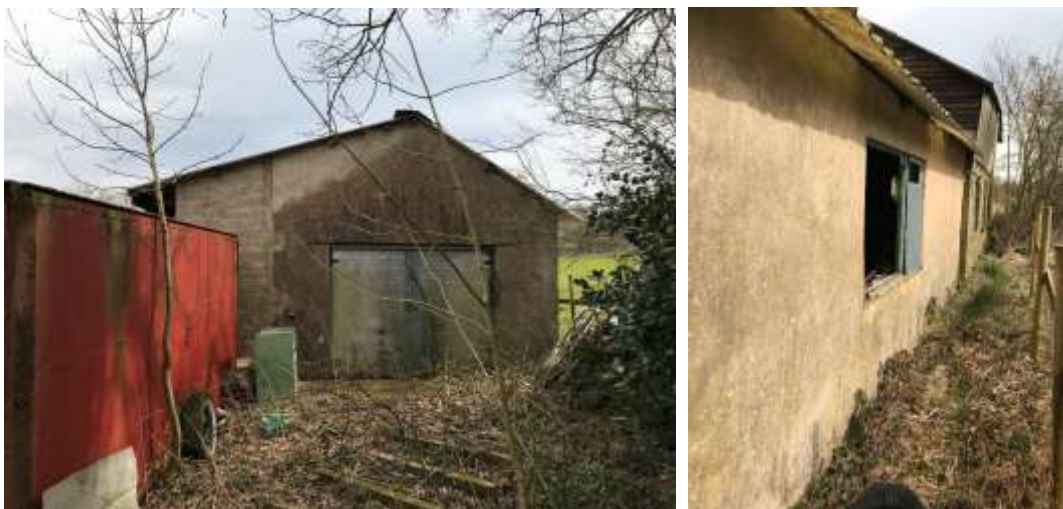
PL. 13. Illustrating cement render finish present to the adjoining agricultural outbuilding to the West and South facing elevation.
