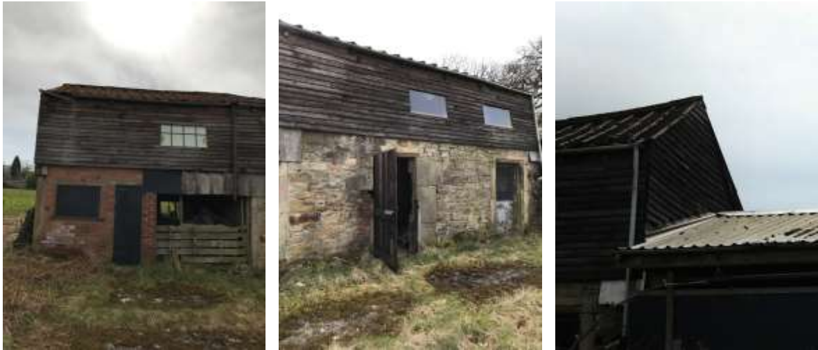
PL. 11. Illustrating low level brick/natural stone claddings and high level horizontal timber boarding to the North Elevation and part of the West facing gable.
