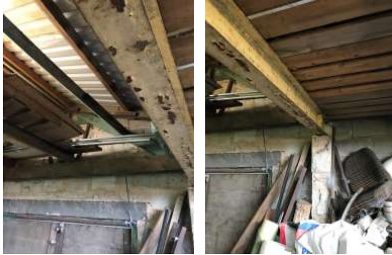
PL. 7. Illustrating section of steel UB currently supported of masonry block piers supporting front North facing section of roof structure over the adjoining agricultural outbuilding structure.
