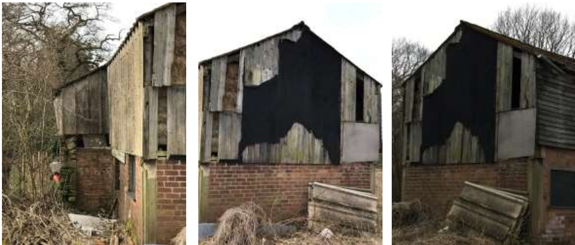
PL. 10. Illustrating low level brick claddings and mixture of high level cement asbestos sheeting and vertical timber boarding to part of the South Elevation and East facing gable.
