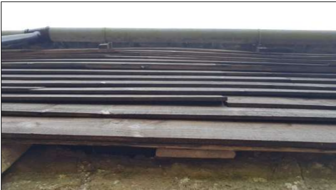
Plate 6: A view of the cladding on the north side of the main barn. The overlapping wooden planks exposed gaps, allowing potential bat access
