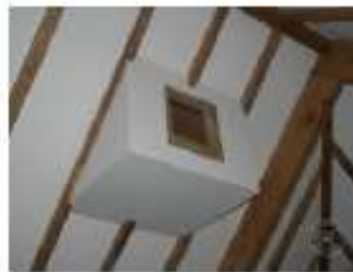
Human access is essential. Here is the interior part of an owl nest space with its insulated inspection panel removed.
