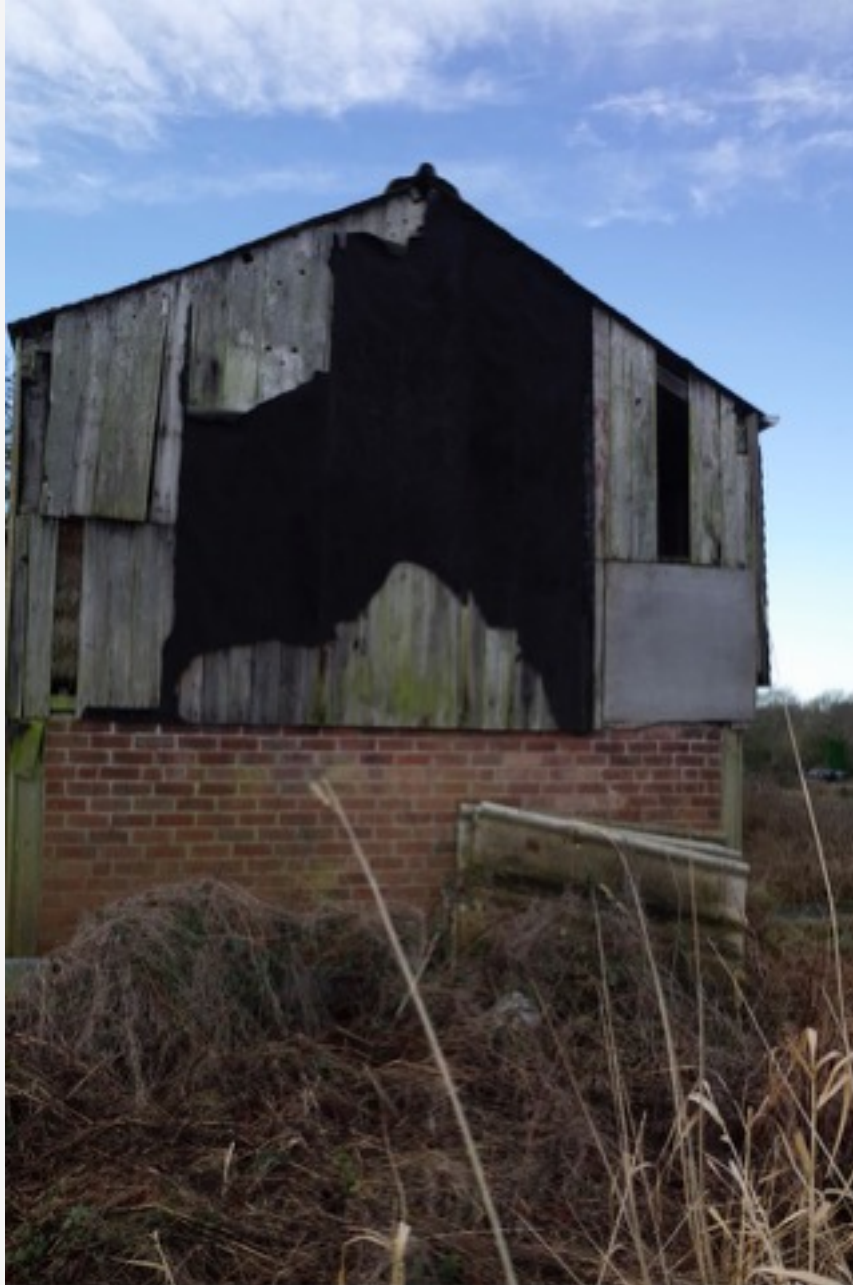
Ruined timber cladding but a solid lower wall
