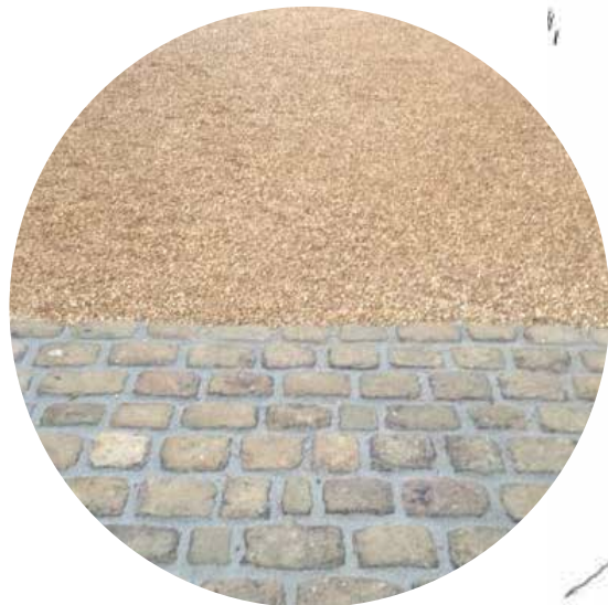
Resin-bound gravel driveways with gritstone rumble strip
